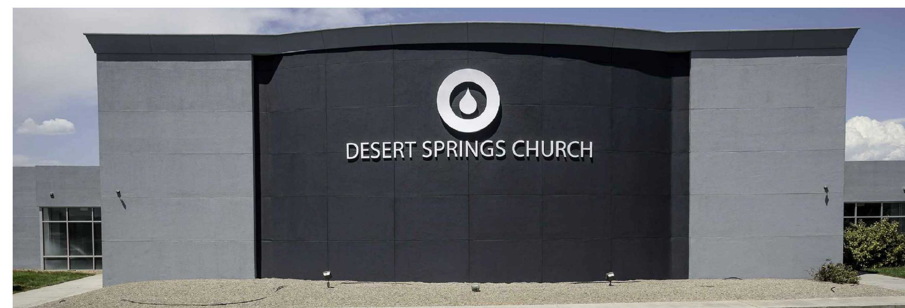
EXISTING SOUTH ELEVATION PHOTO - FOR REFERENCE
