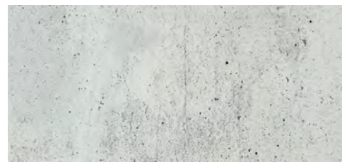
UNFINISHED CONCRETE FLOOR
