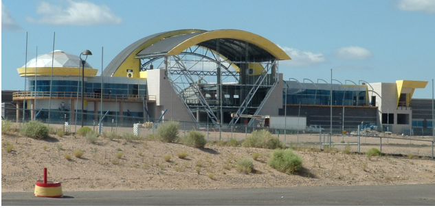
Balloon Museum under construction
