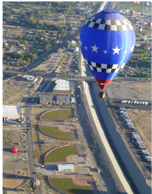
Balloon shown flying over the North Diversion Channel
