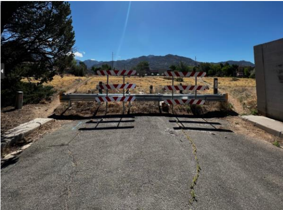
East dead end of existing Sierra Oscura ROW Looking east across Lot #5
