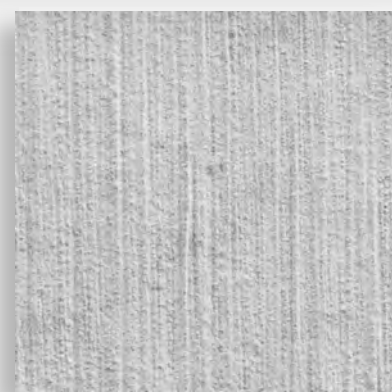
Light Broom Finished TILT-UP CONCRETE WALL EXAMPLE
