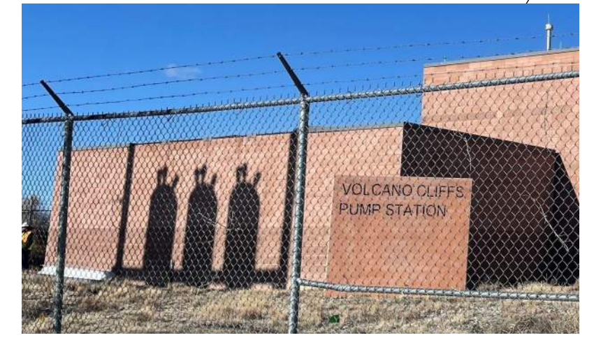
D. EXISTING SURGE TANK ENCLOSURE WALL BEHIND THE PROPERTY SIGN EXISTING PROPERTY SIGN 7'x8' BROWN STUCCO FINISH
