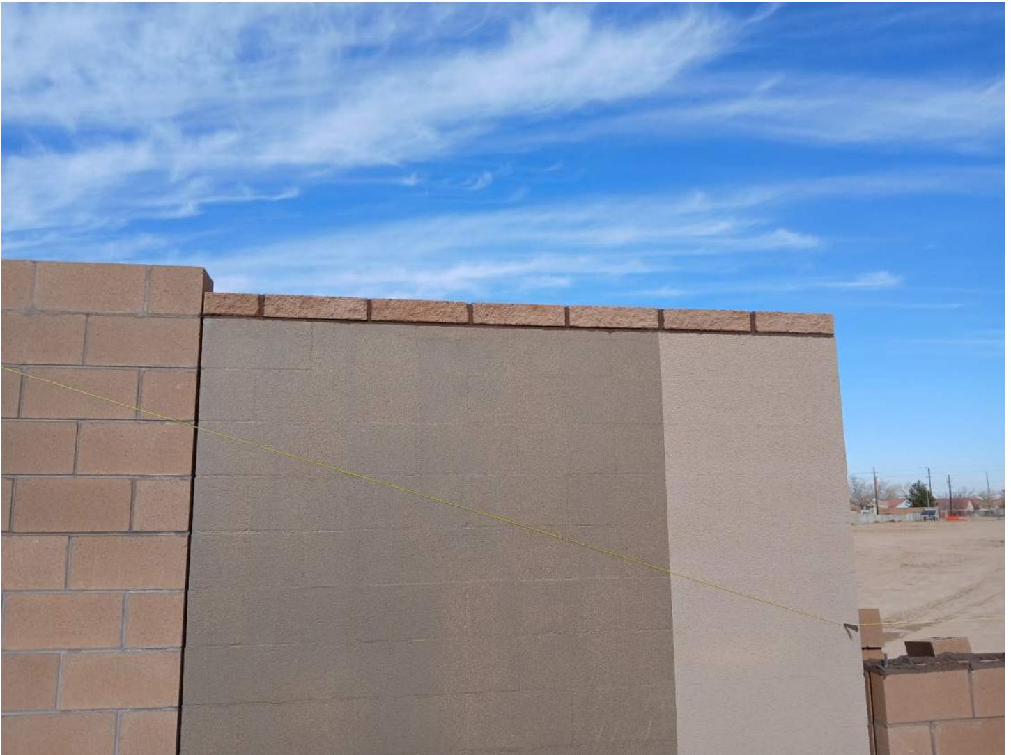
Figure 3 Section of wall with anti-graffiti coating
