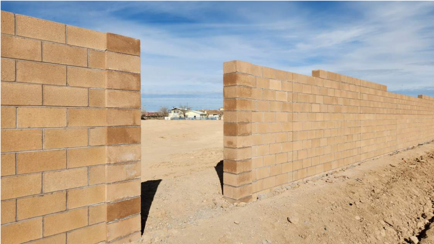
Figure 5 View of pedestrian gate opening with pilasters
