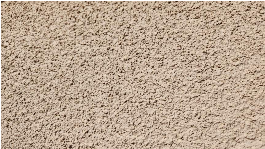
Figure 4 Close up of finished coating
