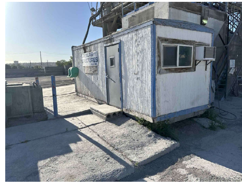
AS-BUILT CONTROL ROOM EXHIBIT PHOTO LOOKING SOUTH EAST
