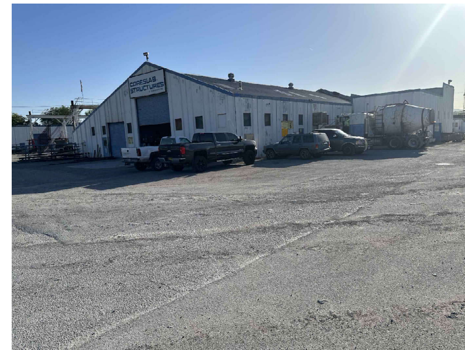
AS-BUILT MAINTENANCE & RECEIVING BUILDING EXHIBIT PHOTO LOOKING NORTH EAST
