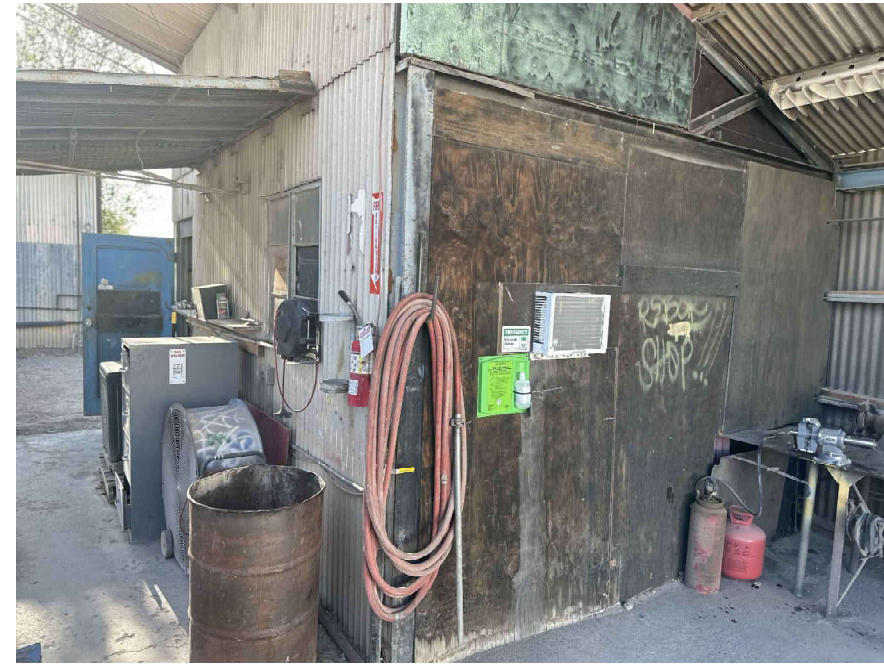
AS-BUILT REBAR FABRICATION BUILDING EXHIBIT PHOTO LOOKING SOUTH EAST
