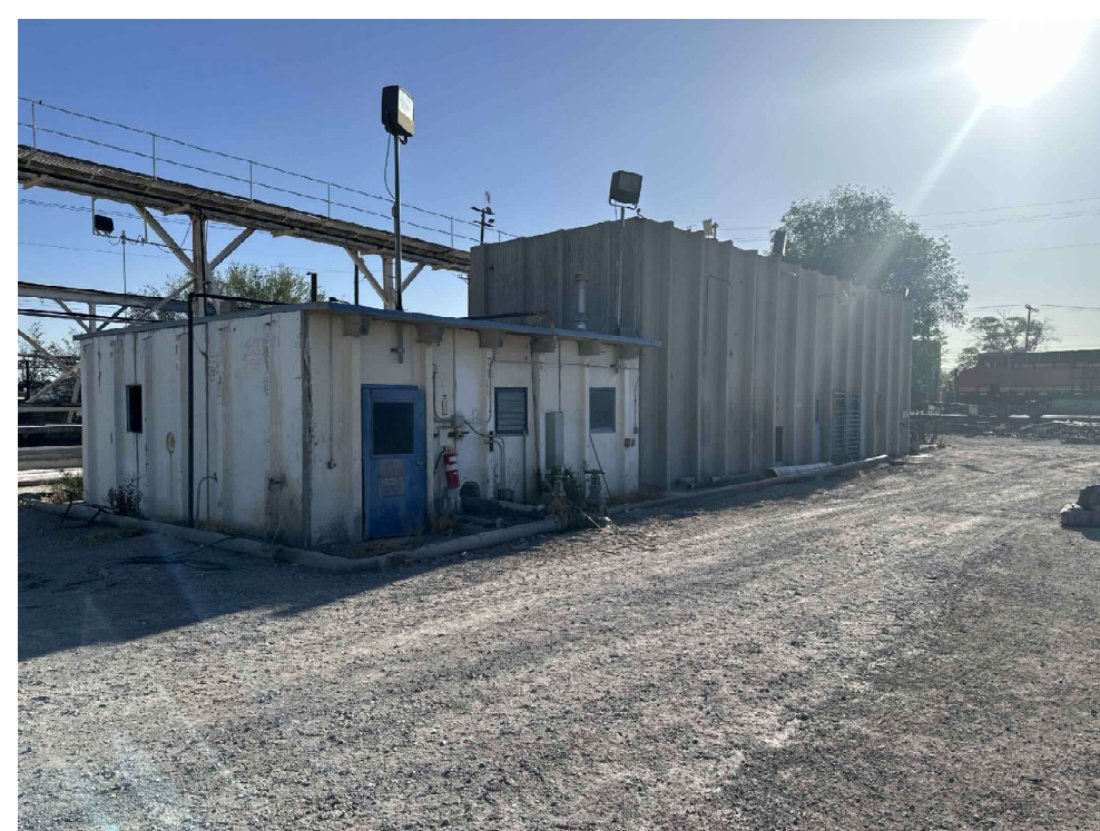
AS-BUILT AS-BUILT QUALITY CONTROL BUILDING EXHIBIT PHOTO LOOKING NORTH EAST
