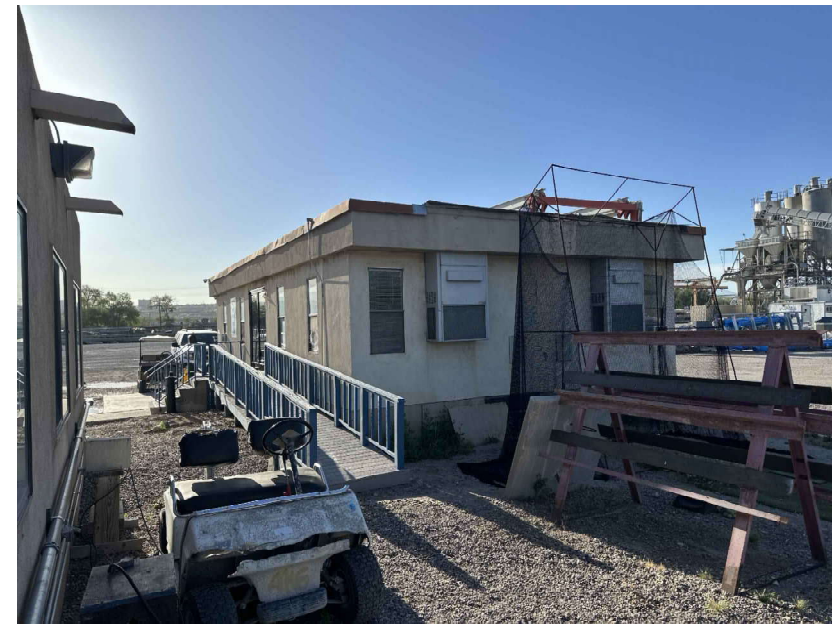
AS-BUILT OFFICE BUILDING EXHIBIT PHOTO LOOKING EAST
