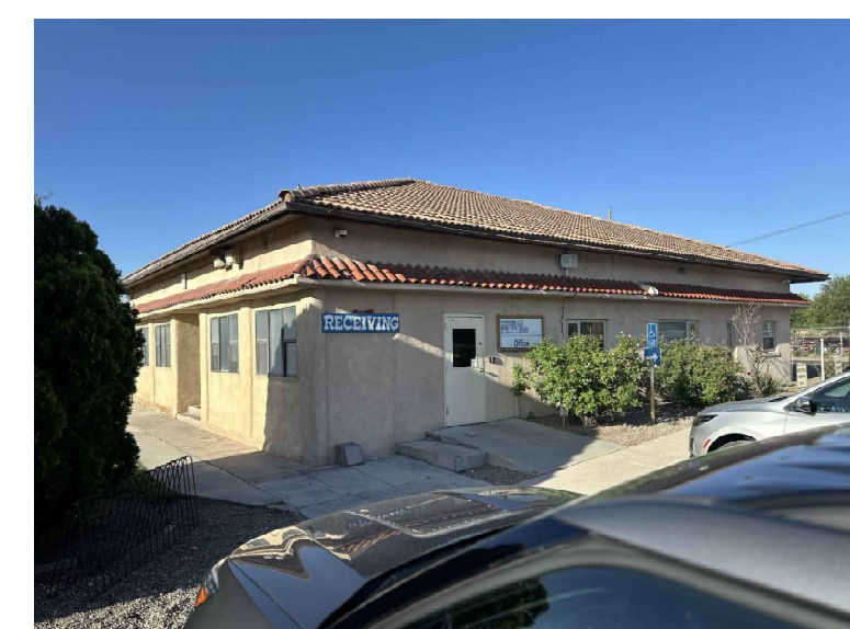
AS-BUILT OFFICE BUILDING EXHIBIT PHOTO LOOKING SOUTH WEST
