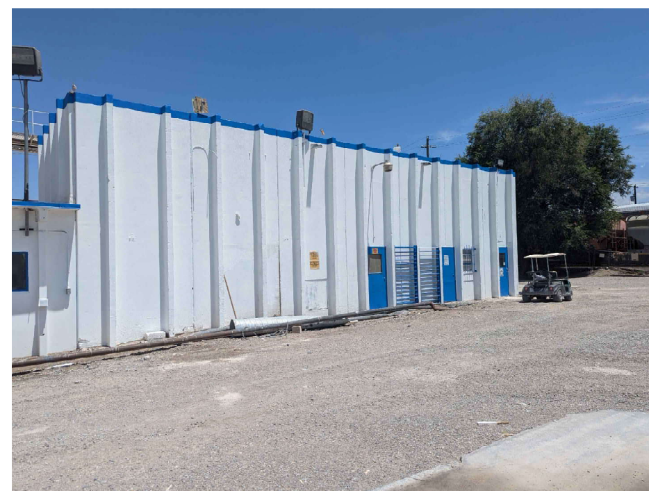
SOUTH ELEVATION: 4 LED FLOOD LIGHTS (14000 LUMENS MAX EA) HEIGHT: 20'
