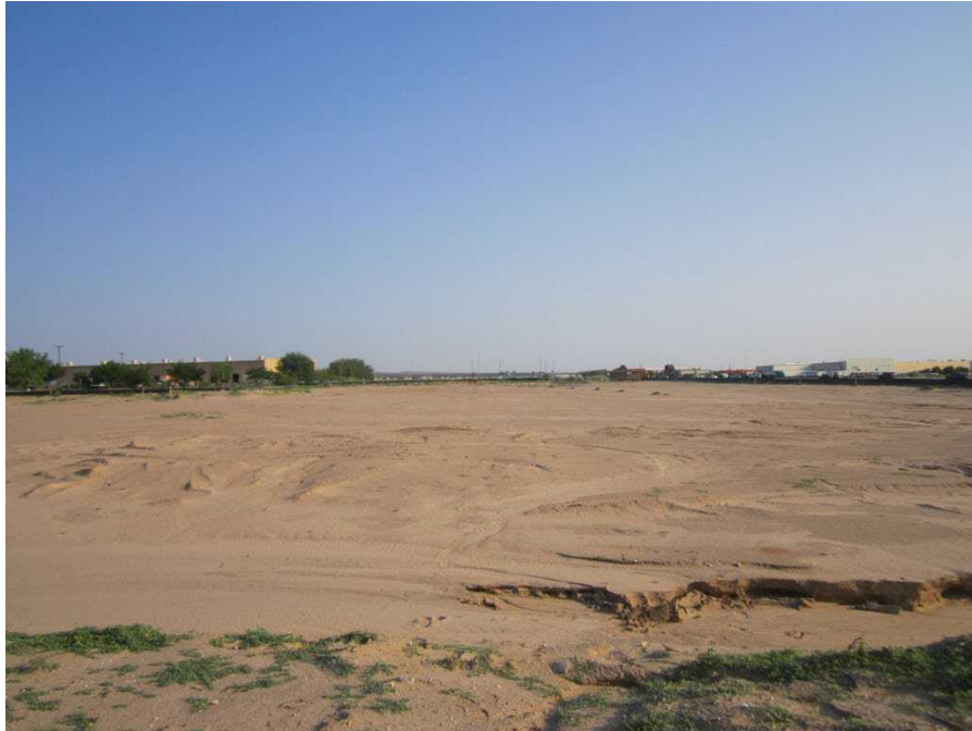
Exhibit 1: View facing north from Bluewater Road of the survey area showing excavation and erosion.
