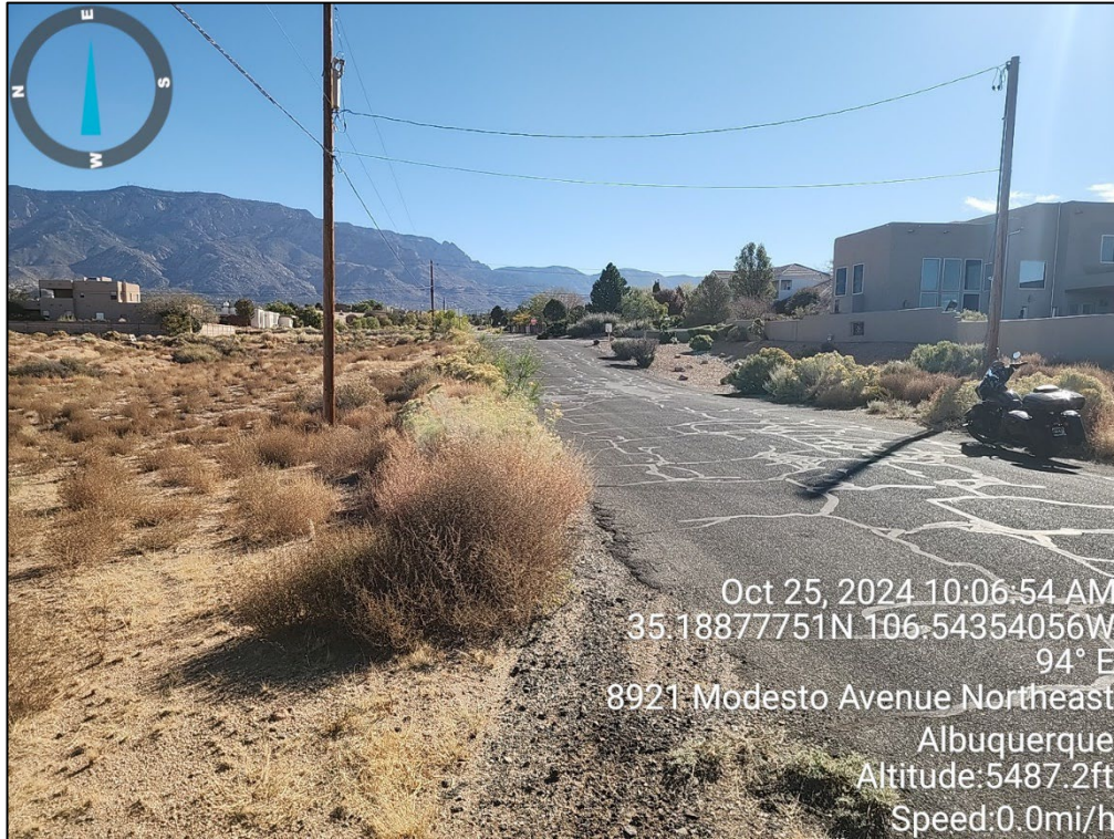
Figure 2 - Lack of Sidewalk on Modesto Ave NE
