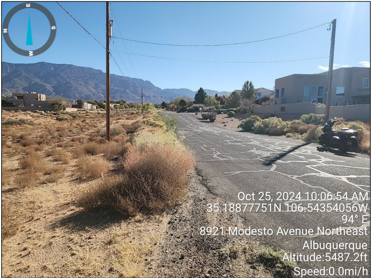
Figure 3 - Lack of Sidewalk on Modesto Ave NE
