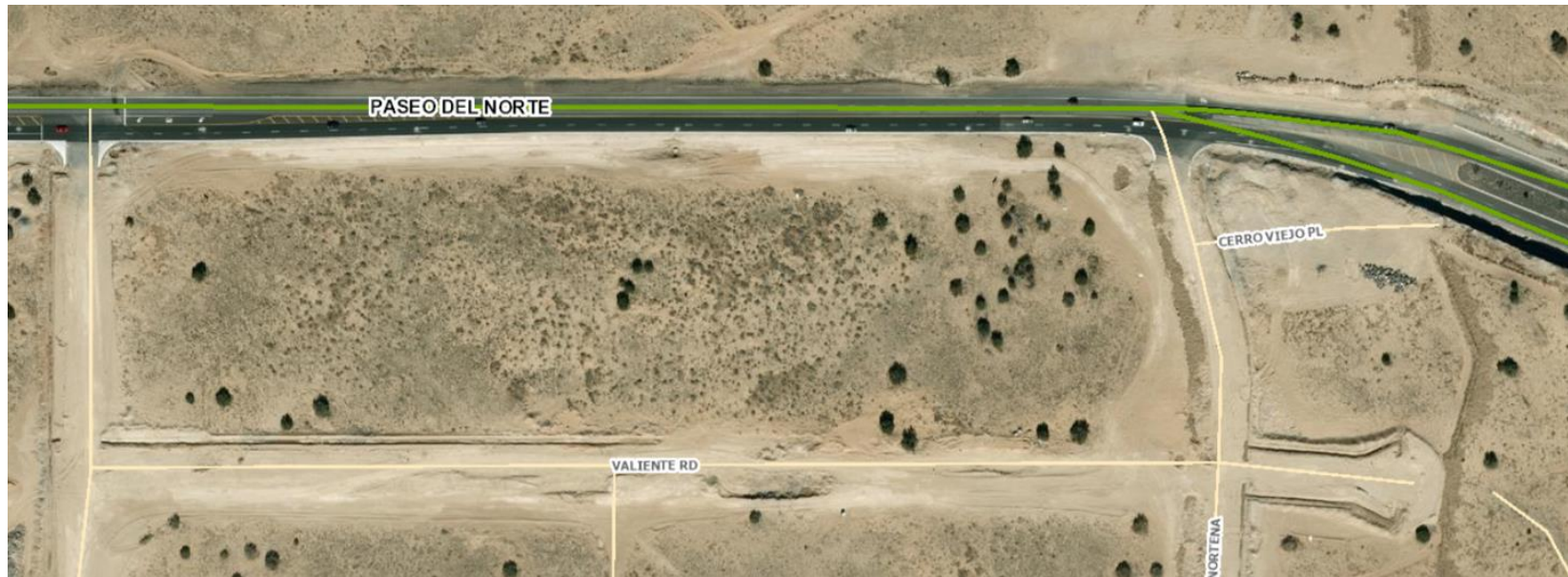
Exhibit C - Exhibit C – 2012–2014: Substantial grading activity along perimeter street corridors.
