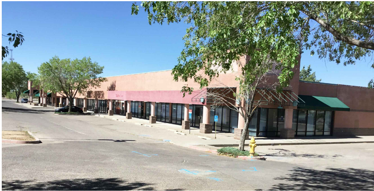
Front of Property Looking Northeast
