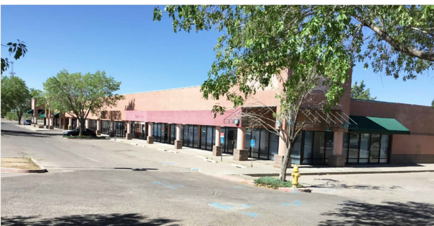
Front of Property Looking Northeast
