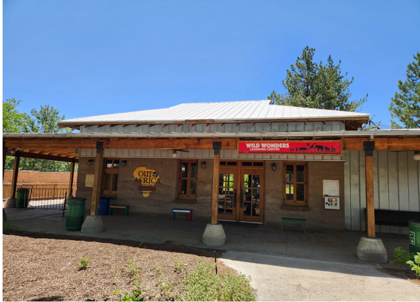
RECENTLY RENOVATED MULTI-PURPOSE BUILDING, KEY OBSERVATION #18
