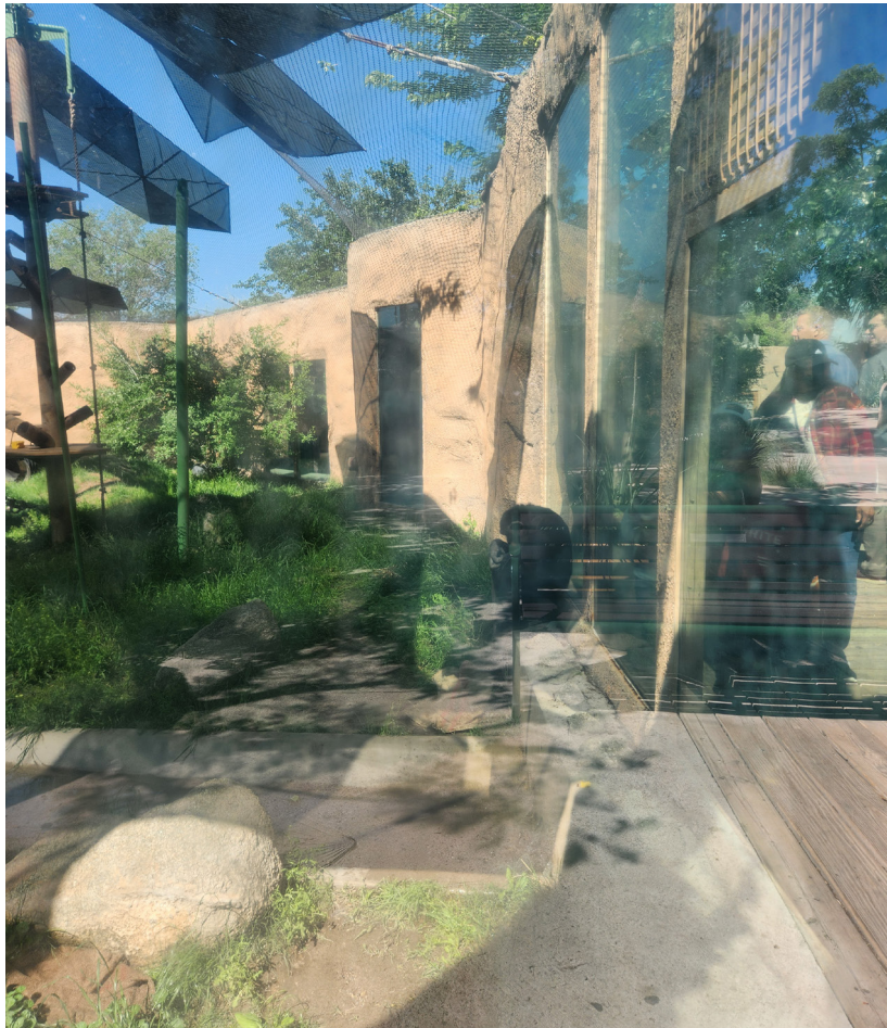
EXISTING MESH-TOPPED CHIMPANZEE HABITAT, KEY OBSERVATION #13
