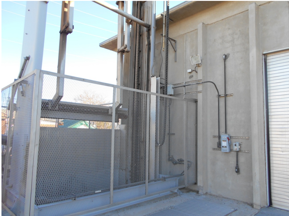
FIGURE 4-1 MECHANICAL BAR SCREEN
