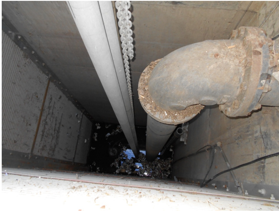
FIGURE 4-5 WET WELL SUMP PUMP
