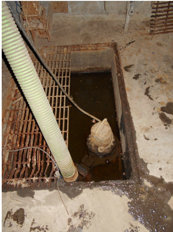
FIGURE 4-7 DRY PIT SUMP PUMP
