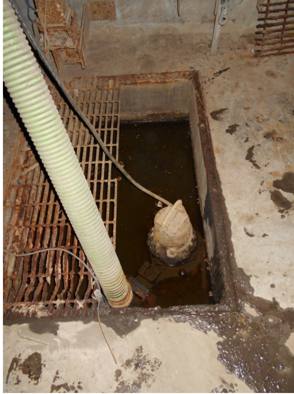
FIGURE 4-7 DRY PIT SUMP PUMP
