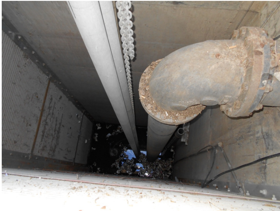
FIGURE 4-5 WET WELL SUMP PUMP
