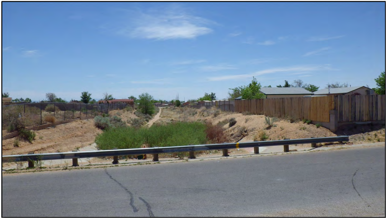
Photo 26: Looking south from Vancouver Road down the existing earthen channel.
