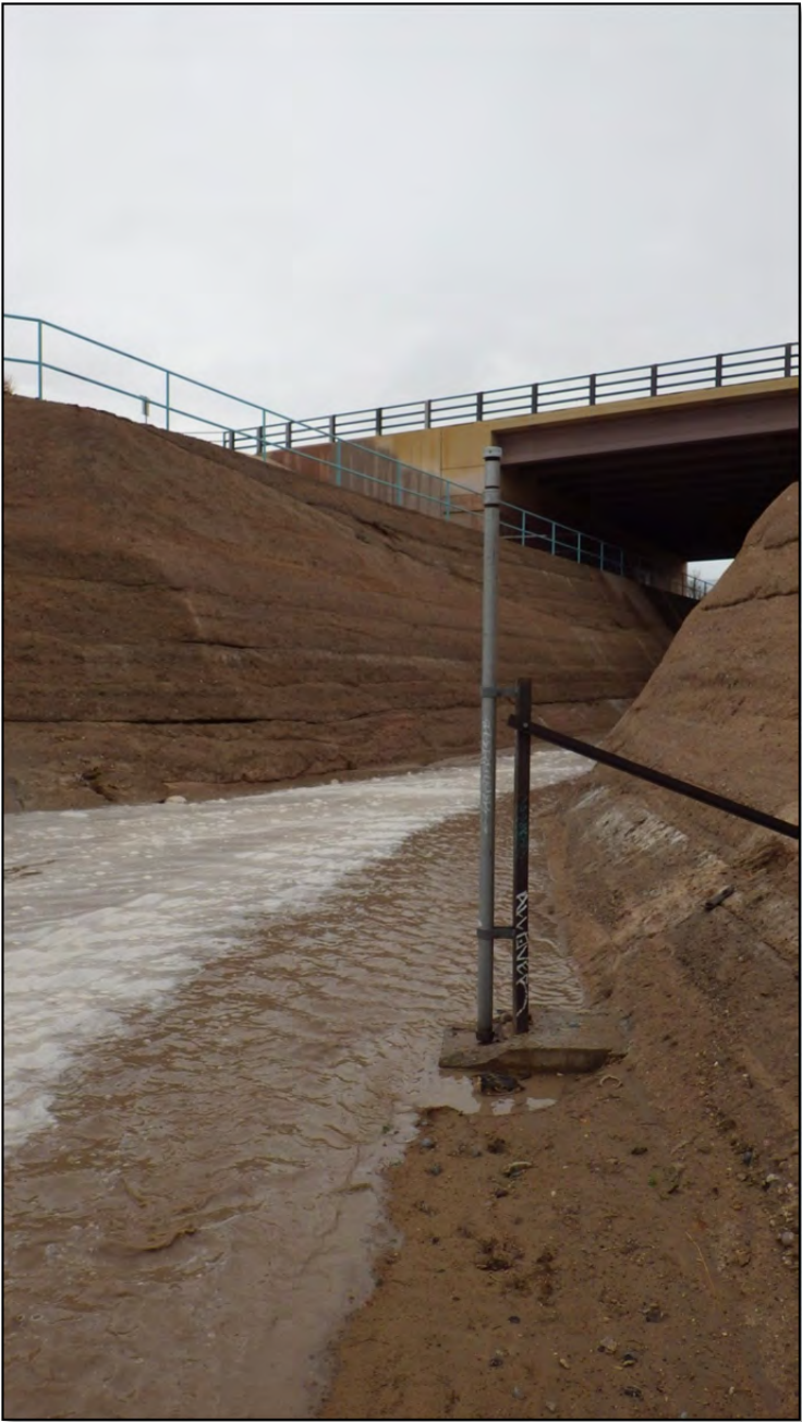
Photo 13: Stream gauging station at the outlet structure of Swinburne Dam; the gauge is located in the 2-inch galvanized steel pipe on the right.
