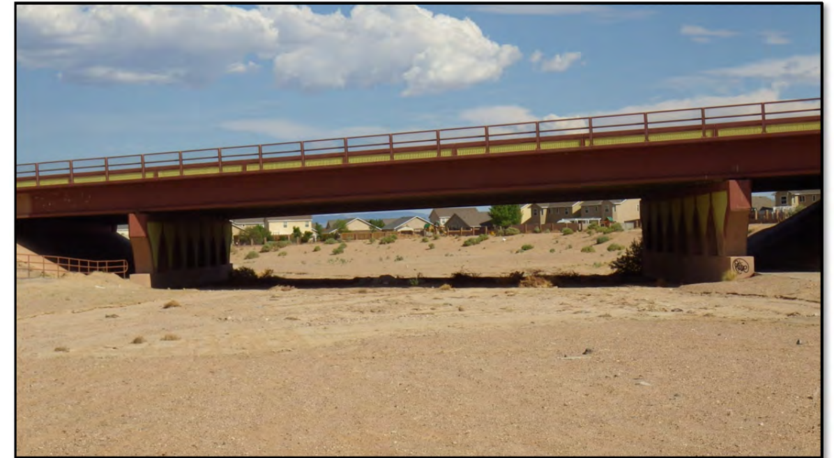
Photo 8: McMahon Blvd Bridge crossing of the Calabacillas Arroyo, looking upstream.
