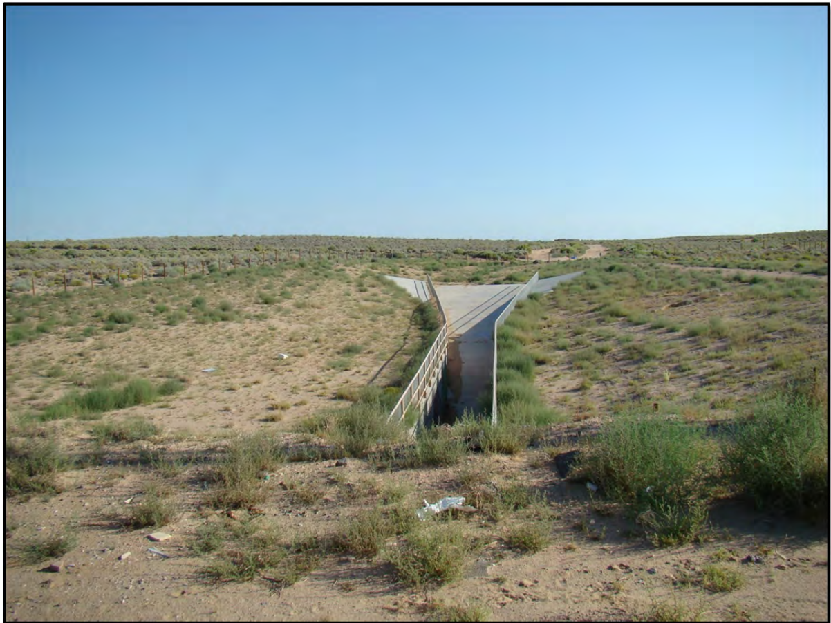
Photo 6: Inlet to the Saltillo storm drain.
