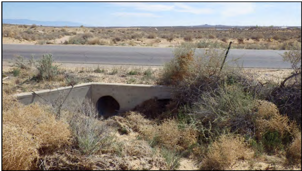
Photo 31: Culverts at Southern Blvd & Tributary D (2 – 24” CMP, capacity ≈ 24 cfs).
