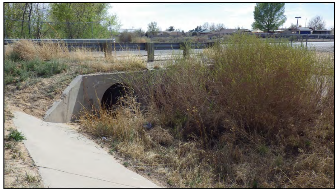
Photo 24: Rainbow Tributary crossing at Pecos Loop (4 – 48” CMP, capacity ≈ 333 cfs).
