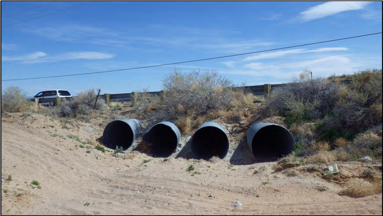
Photo 29: Tributary B crossing at Southern Blvd (4 – 48” CMP, capacity ≈ 232 cfs).
