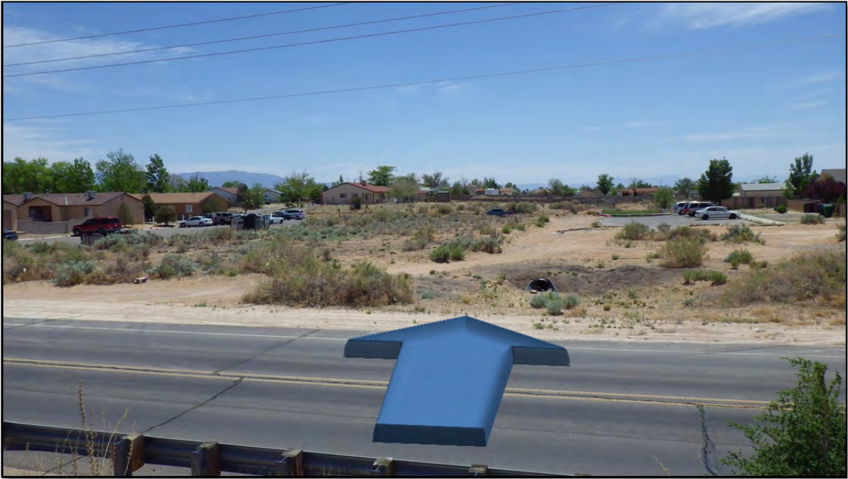
Photo 23: Looking south from Tulip Road. Except for one 18" CMP culvert, no drainage infrastructure exists between Tulip and Vancouver Roads.; apartment buildings on both sides are in the 100-year floodplain
