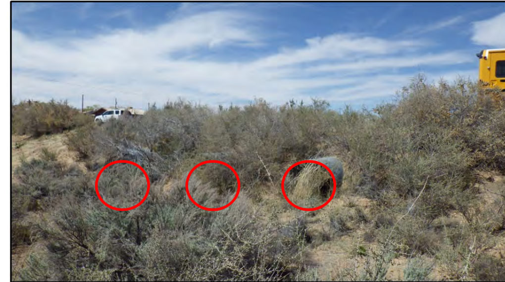
Photo 34: Looking upstream at the Tributary P crossing at Northern Blvd (3 – 48" CMP, capacity ≈ 258 cfs).
