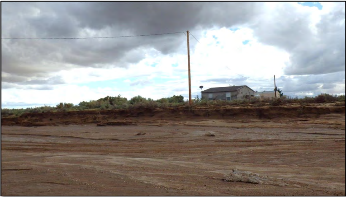
Photo 27: House near the east bank of the Calabacillas Arroyo upstream of Northern Blvd.
