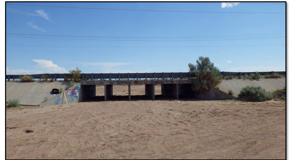
Photo 9: Concrete box culverts at Southern Blvd, looking downstream.
