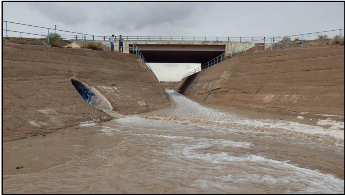
Photo 5: Swinburne Dam, looking upstream at the outlet structure.
