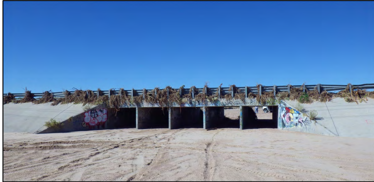
Photo 20: Southern Blvd. Crossing of the Calabacillas Arroyo, looking upstream.
