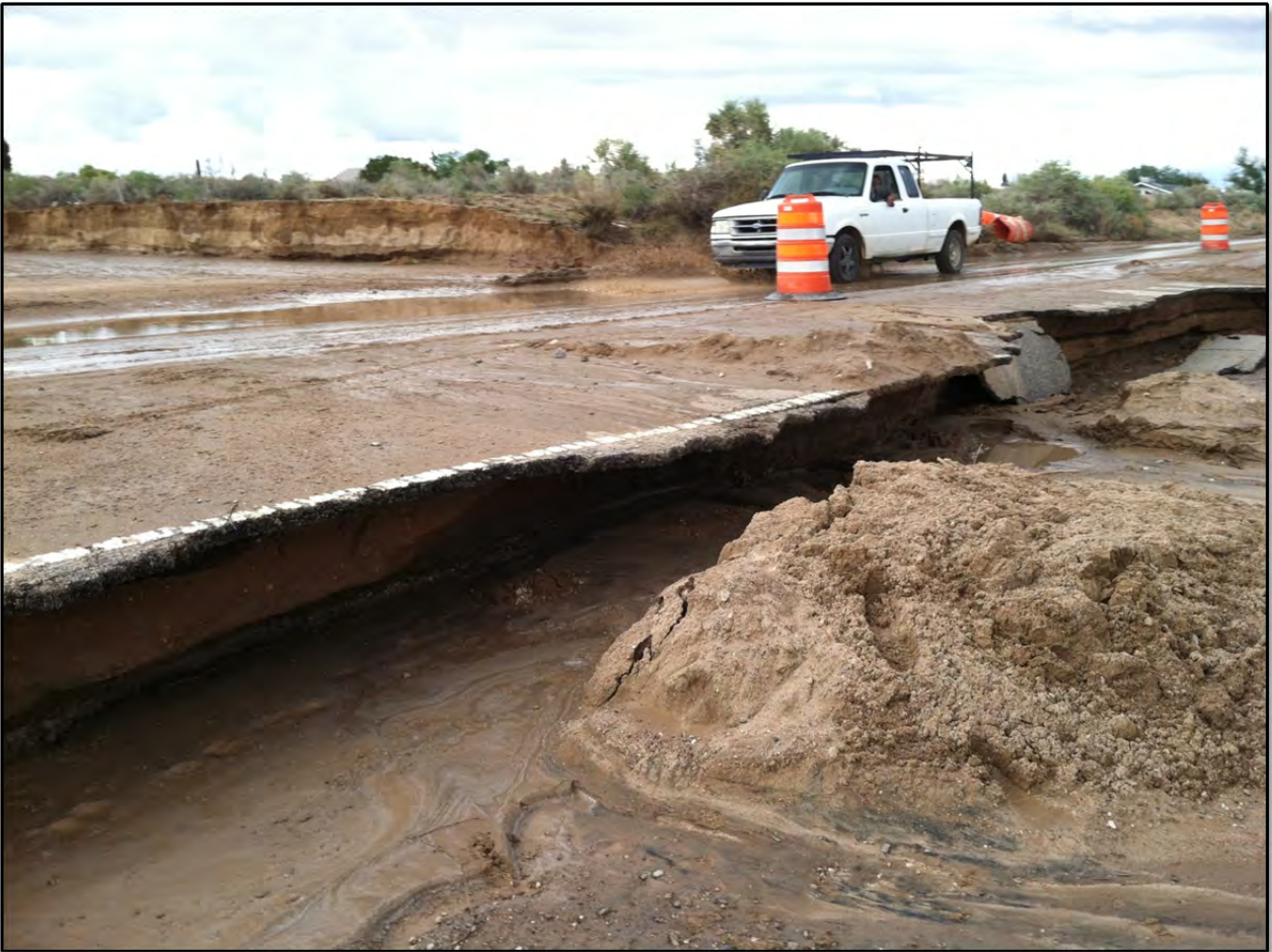
Photo 19: The south lane of Northern Blvd is partially undermined following the storm of September 13, 2013.
