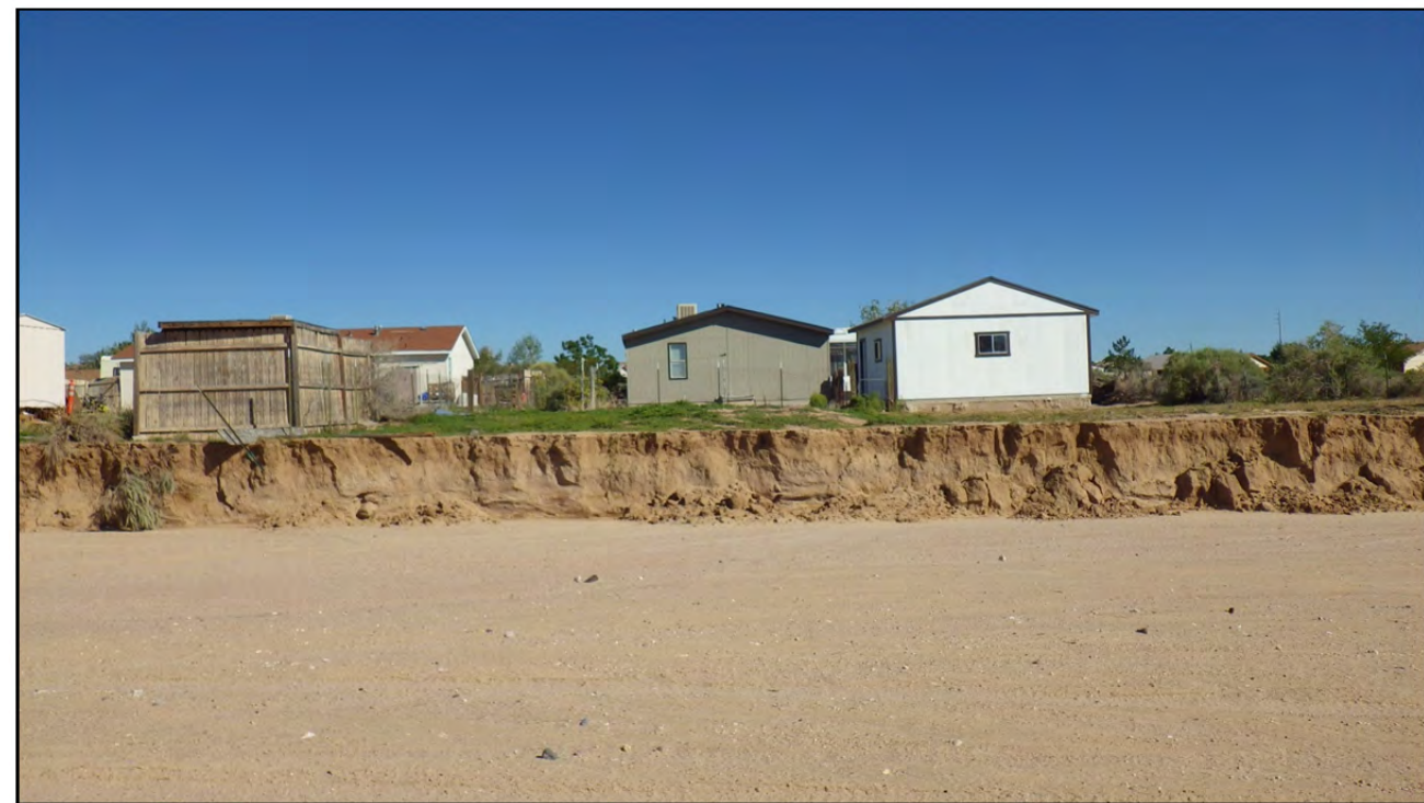
Photo 28: Houses on the east bank of the Calabacillas Arroyo north of Southern Blvd threatened by bank erosion.
