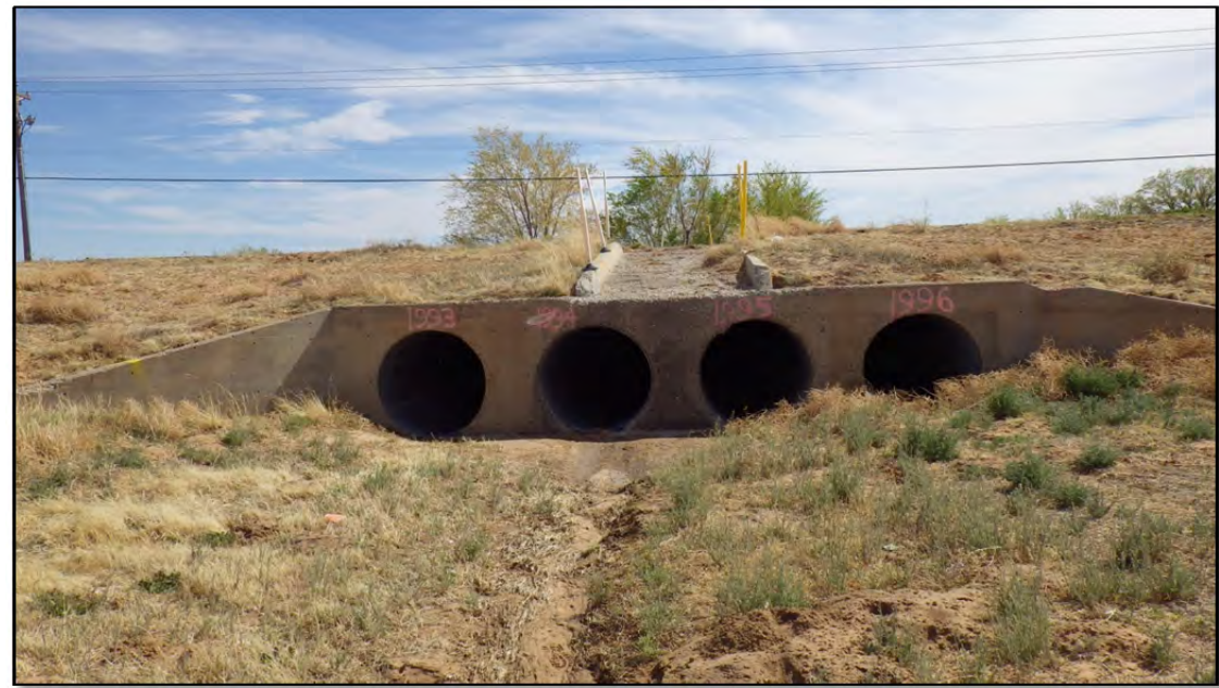
Photo 25: Rainbow Tributary crossing at Southern Blvd (4 – 48” CMP, capacity ≈ 438 cfs).
