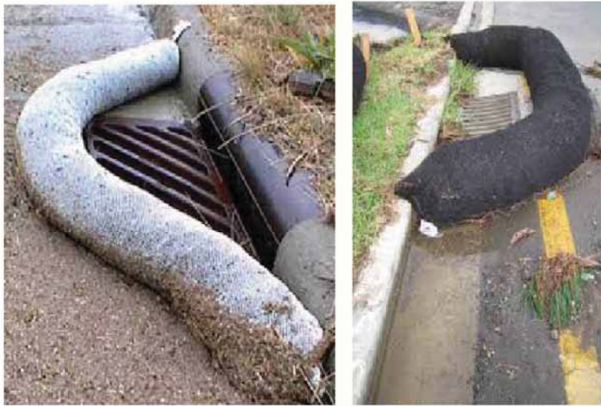
Curb Storm Inlet Protection with Wattles
