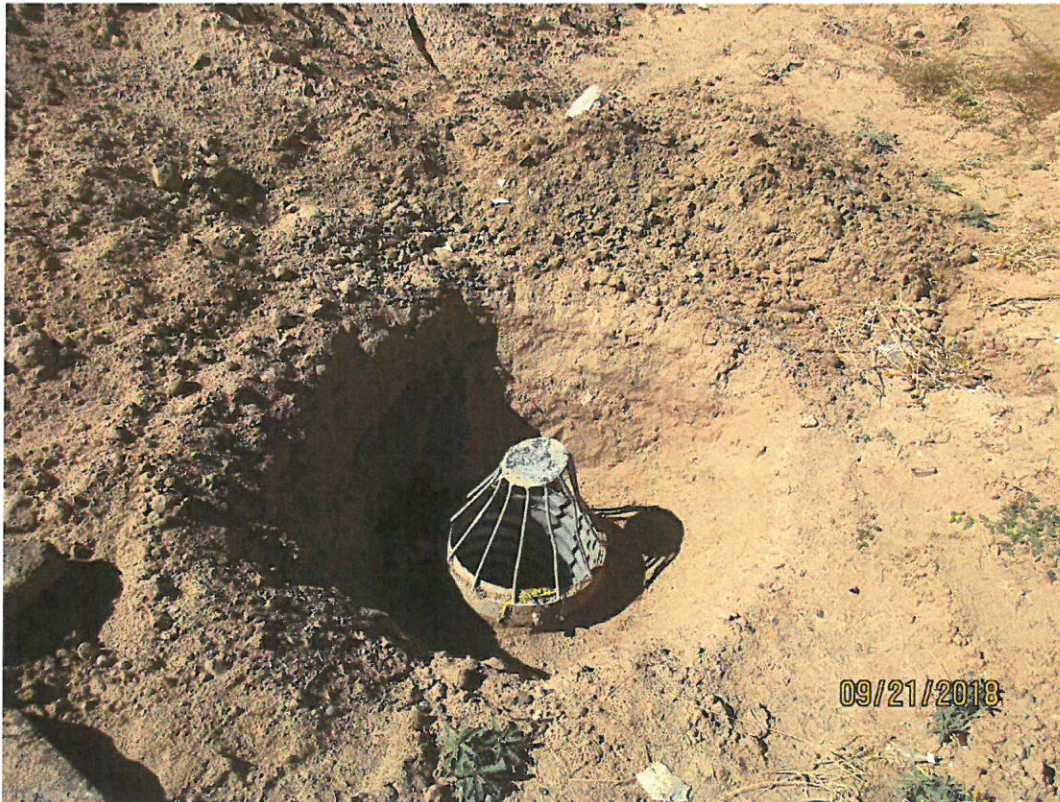
Drainage inlet requires protection.
