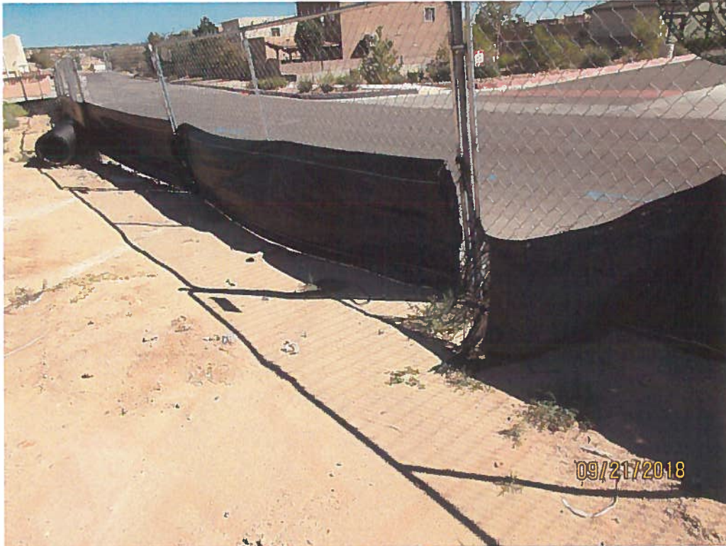
Silt fence gap and silt fence is torn.
