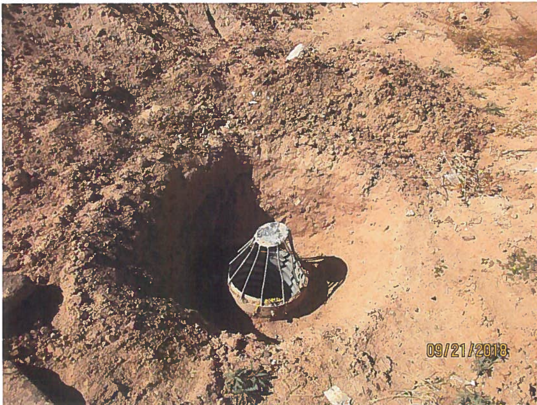
Drainage inlet requires protection.
