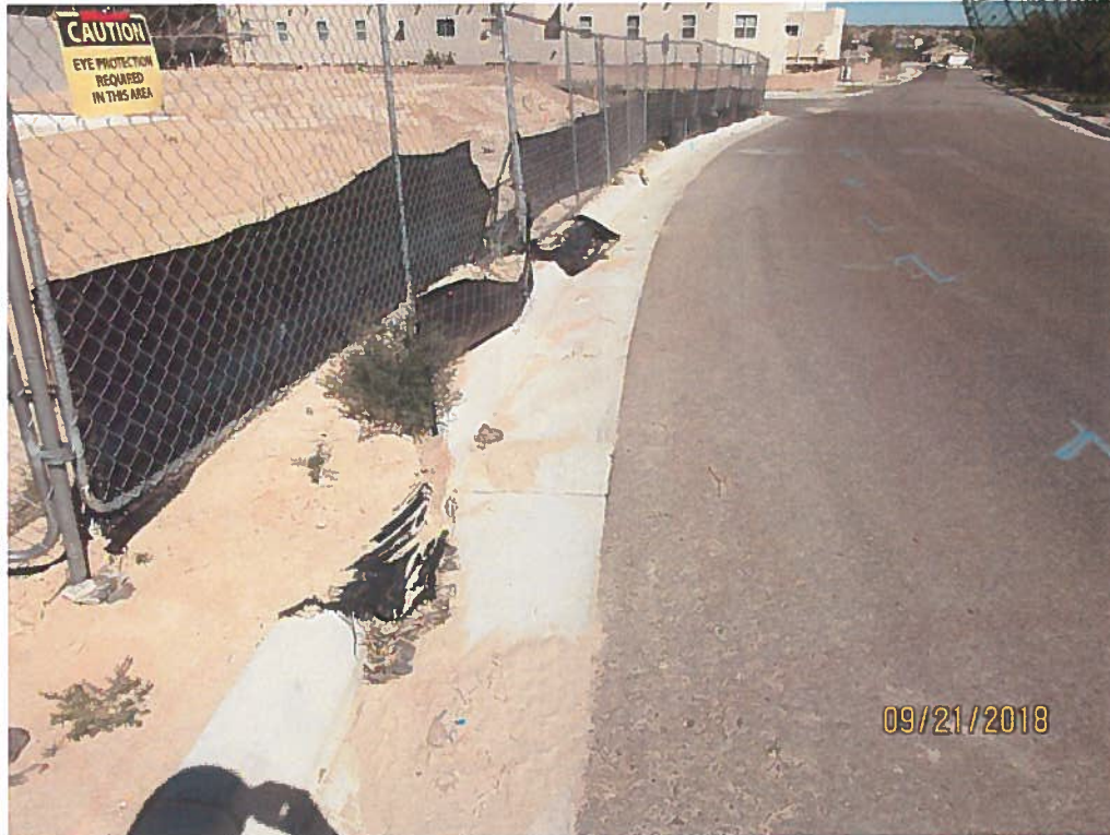
Silt fence bulging, too much dirt behind silt fence and sediment in the gutter.
