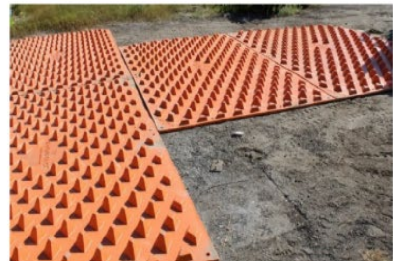
INSTALL FODS ACCORDING TO THE MANUFACTURER'S SPECIFICATIONS. FODS TRACK-OUT CONTROL MATS CAN BE USED WITH A STABILIZED CE OR ALONE, AS LONG AS THEY CAN ACCOMMODATE THE TURNING MOVEMENTS OF THE LARGEST VEHICLES EXITING THE SITE.
