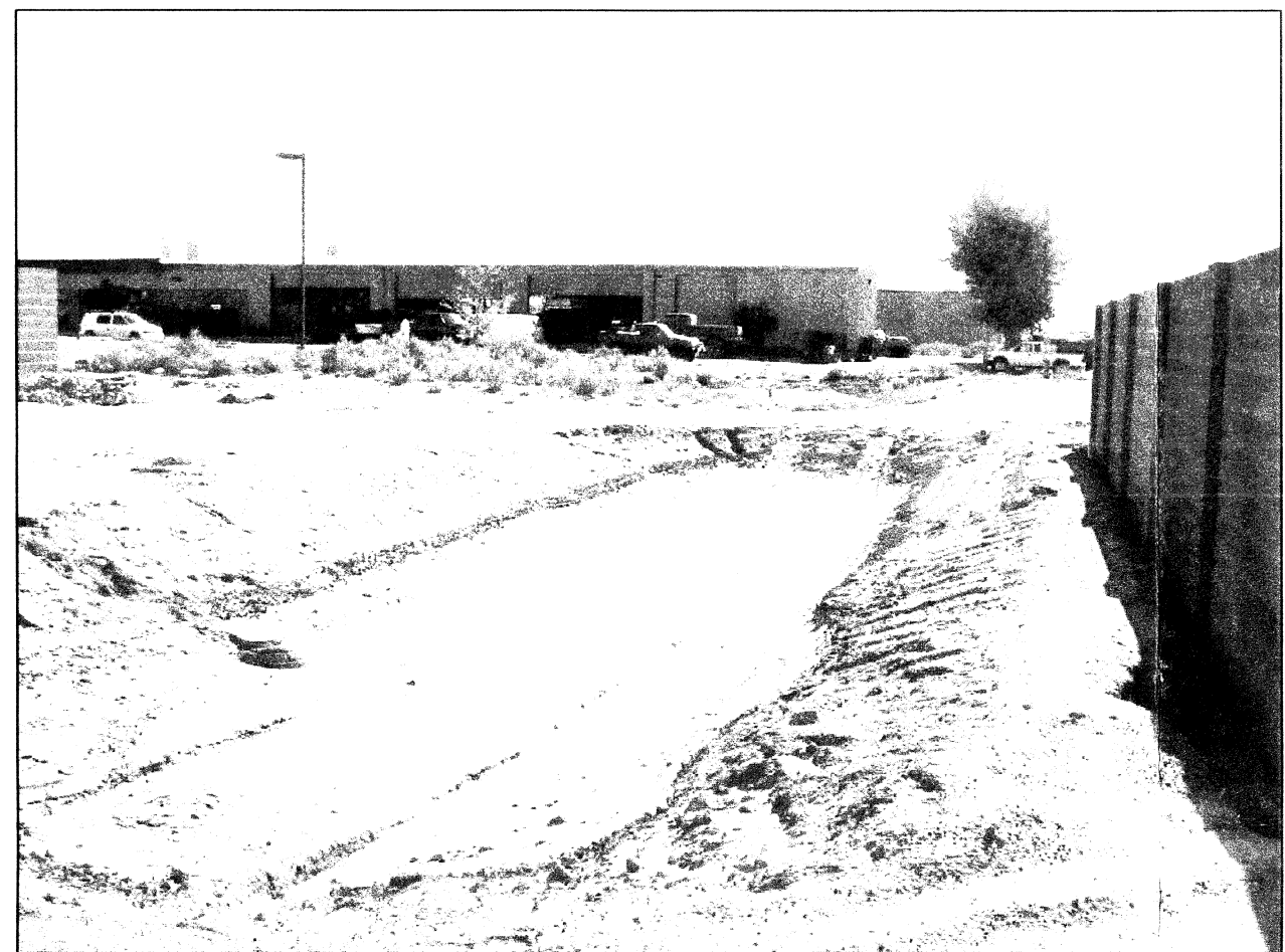
I: POND WILL ACCEPT FLOW FROM SITE CURRENTLY UNDER CONSTRUCTION. POND DOES NOT APPEAR TO BE COMPLETED, BUT LOOKS LIKE IT WILL BE PERMANENT, FUNCTION PROPERLY, AND OF ADEQUATE SIZE.
