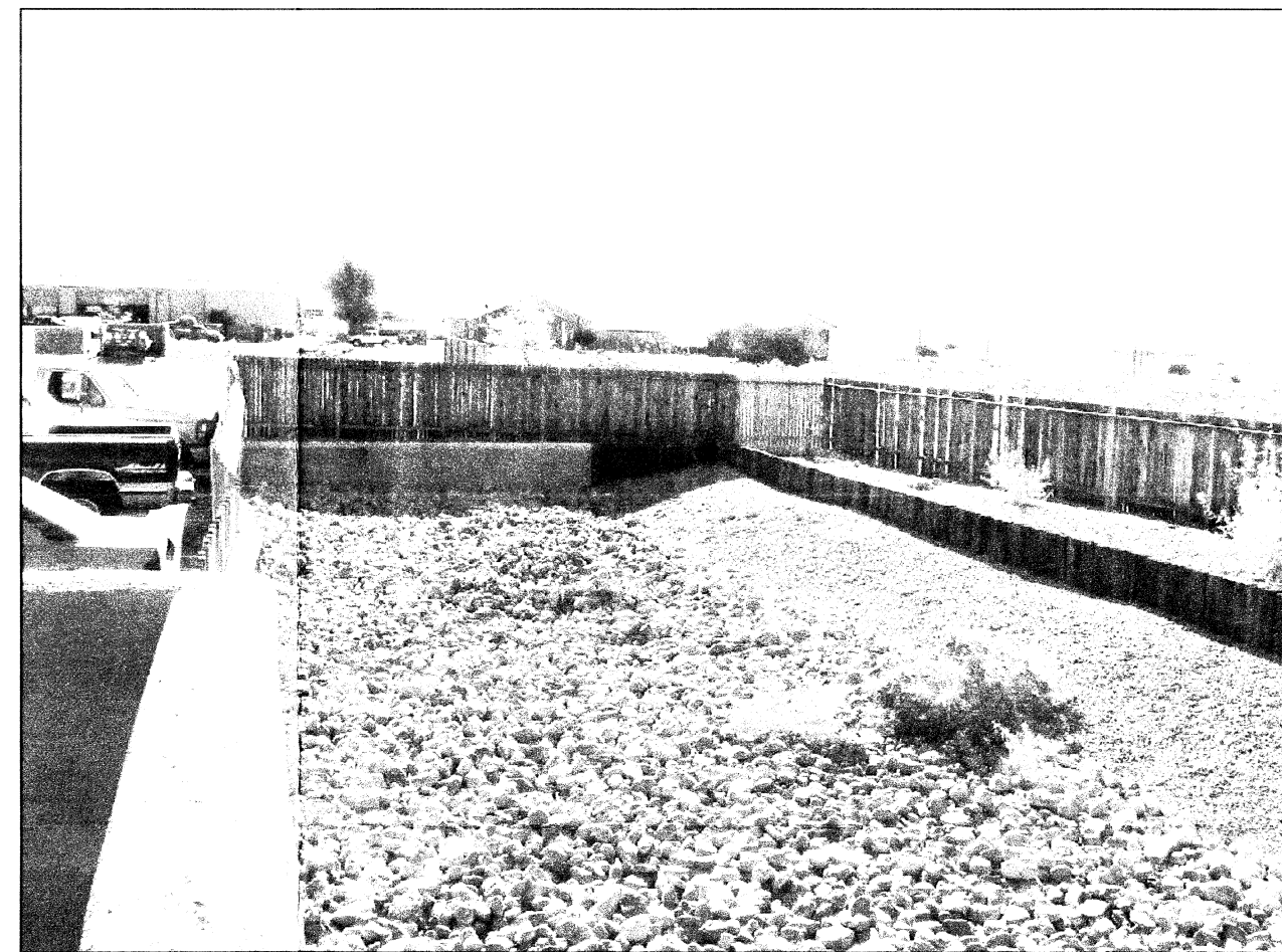
G: ACCEPTS FLOW FROM BARBER SHOP AND OFFICES, SE CORNER SOUTHERN AND 21ST. POND APPEARS TO BE PERMANENT, FUNCTIONING PROPERLY, AND OF ADEQUATE SIZE.
