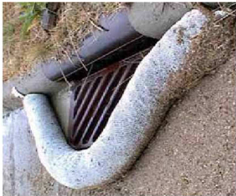
Curb Storm Inlet Protection with Wattles
