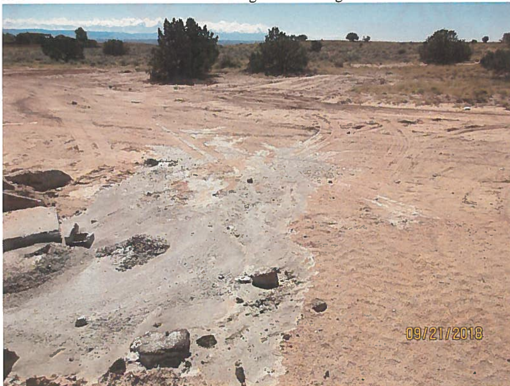
Wash-out and construction debris on lot west of project. Area disturbed outside project boundaries.
