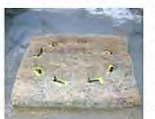
3. Position the mat. Place Inlet Filter on grate with the net side down, flush to the back edge and extending beyond the grate opening on the front and both sides. The zip ties attach Inlet Filter to the inlet grate cover WITHOUT LIFTING THE GRATE COVER.
