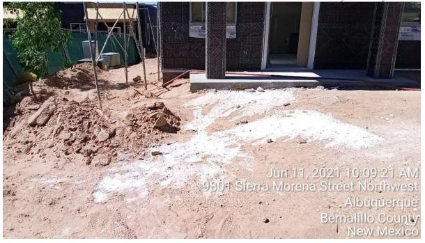
6. Inactive portions of the site have not been stabilized in accordance with CGP 2.2.14 (1<sup>st</sup> Violation). The pond on Lot 12A has been relocated to lot 11B and has been inactive for a long time. Construction support activities disturbed a portion of the neighbor's lots 9A, 9B, 10B, and 12B. You may have to pay that neighbor for the use of his property. Stabilization of that property will be the responsibility of this site unless the neighbor obtains NPDES permit coverage.
