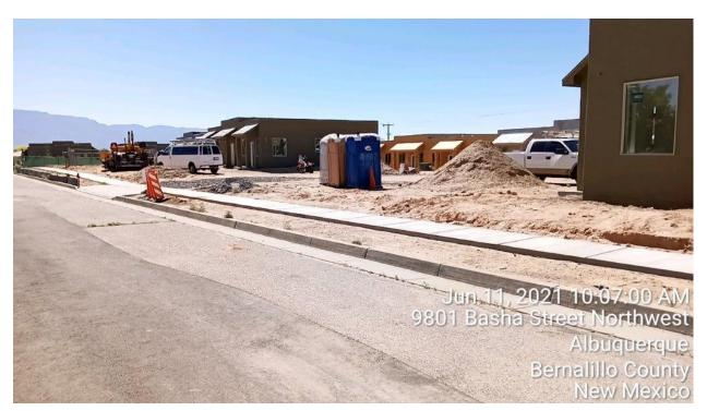
4. Sediment has accumulated greater than half the height of the silt fence along Buglo Street (1st Violation)
