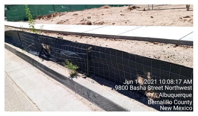
3. Install perimeter silt fences as shown in the ESC Plan (1st Violation)
