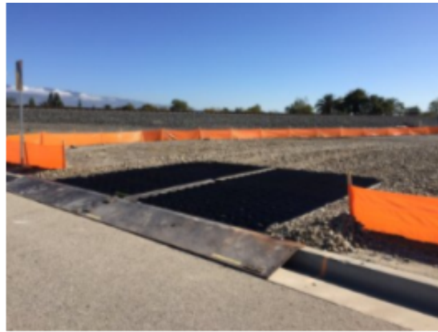
SEDIMENT TRACK OUT CONTROL
