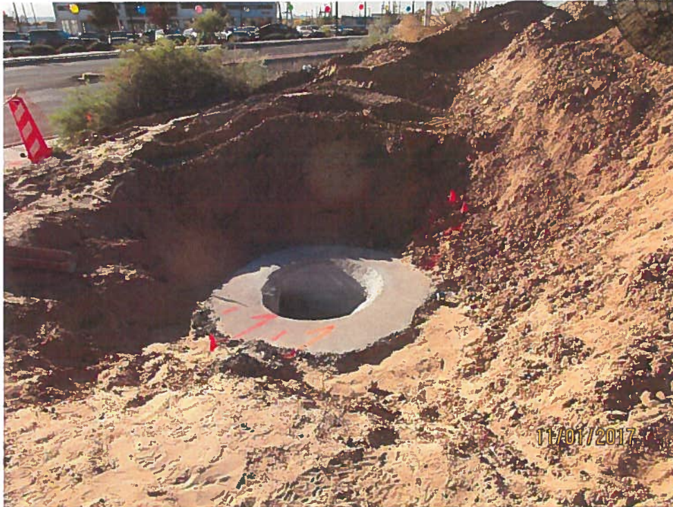
Opening into storm drain system with no BMP.
