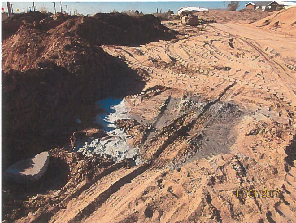
One of two concrete wash-outs.
