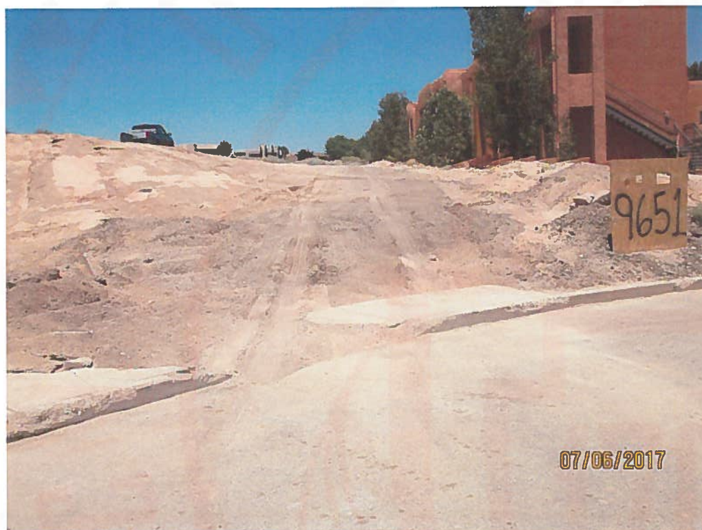
No track-out pad. Also, long and steep area with no sediment BMP.
