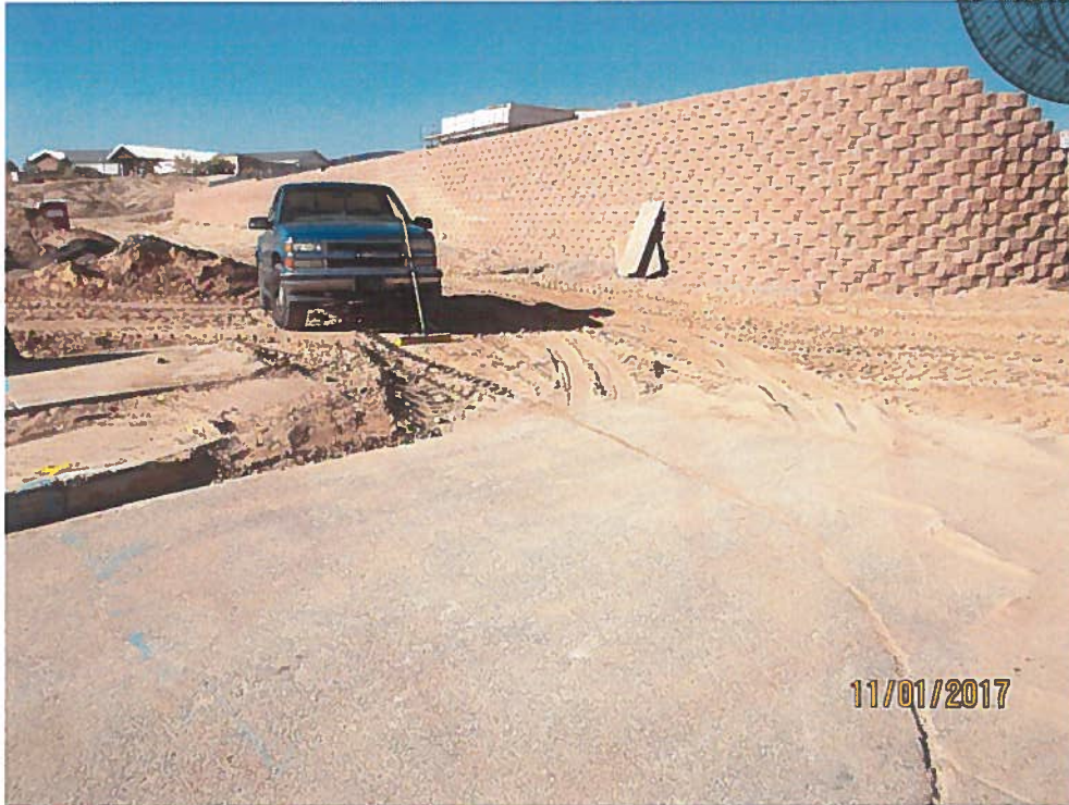
No sediment BMP at asphalt interface.
