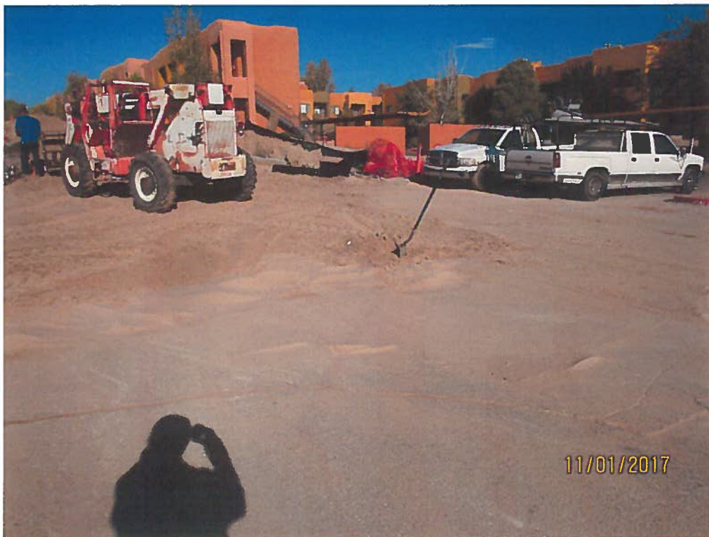
No sediment BMP at asphalt interface.
