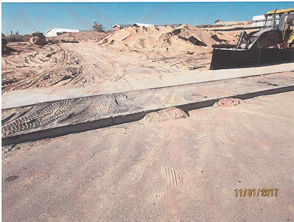
No track-out pad. Sediment in access road.
