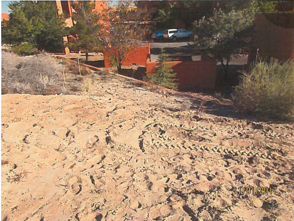
Disturbed area in northwest corner without a sediment BMP.
