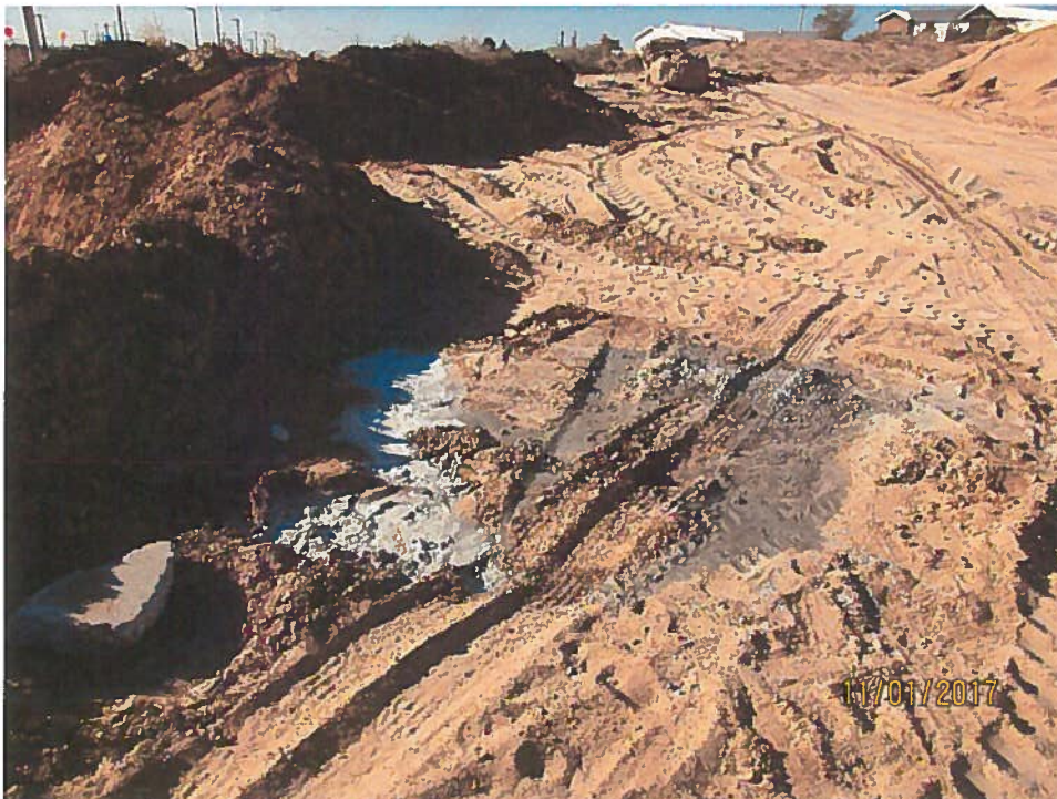
One of two concrete wash-outs.
