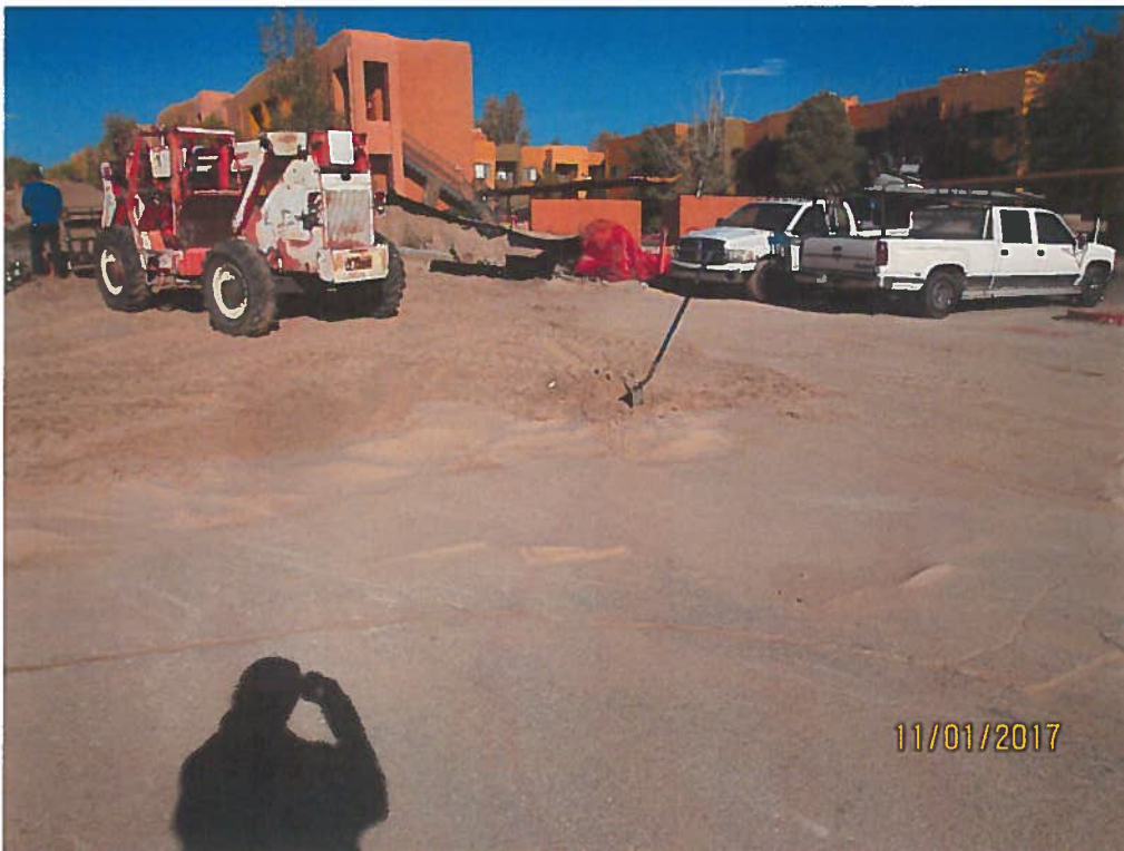
No sediment BMP at asphalt interface.
