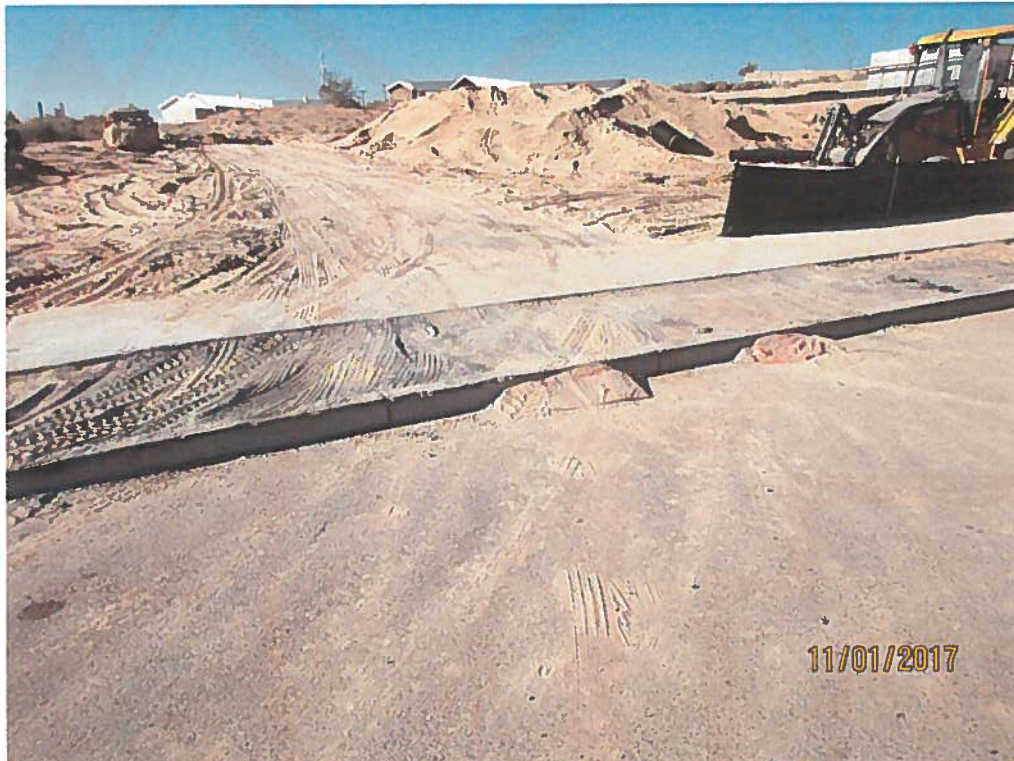
No track-out pad. Sediment in access road.
