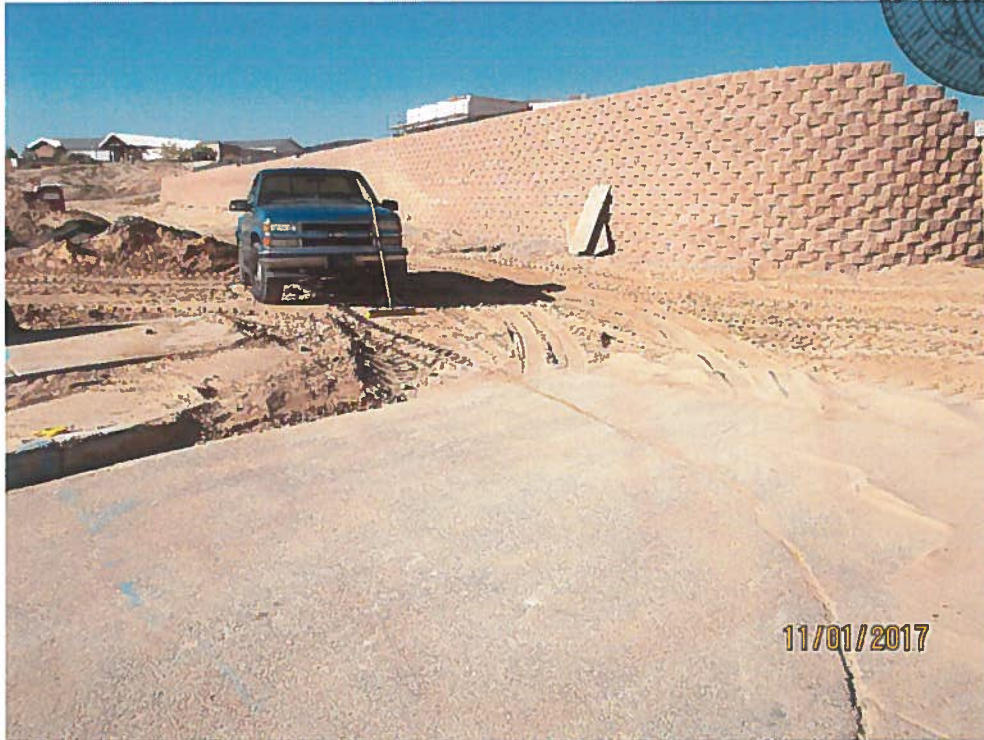
No sediment BMP at asphalt interface.
