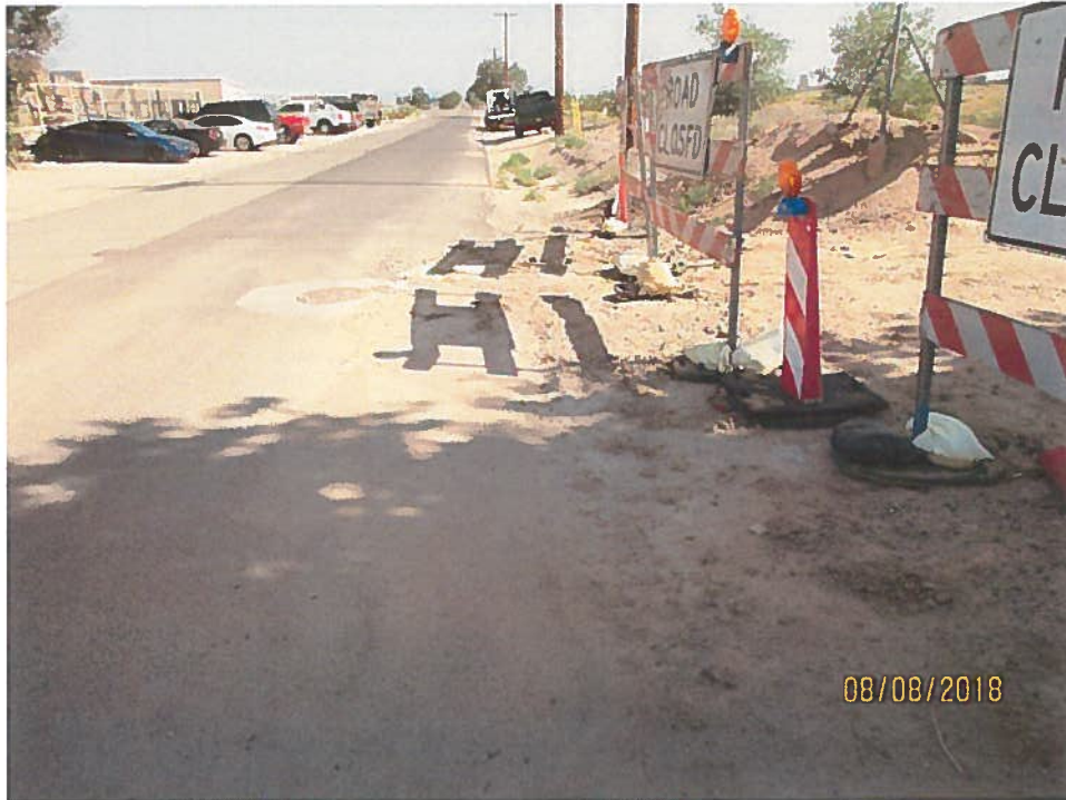
Sediment in San Pedro Blvd. Partial sediment BMP for a portion at San Pedro.
