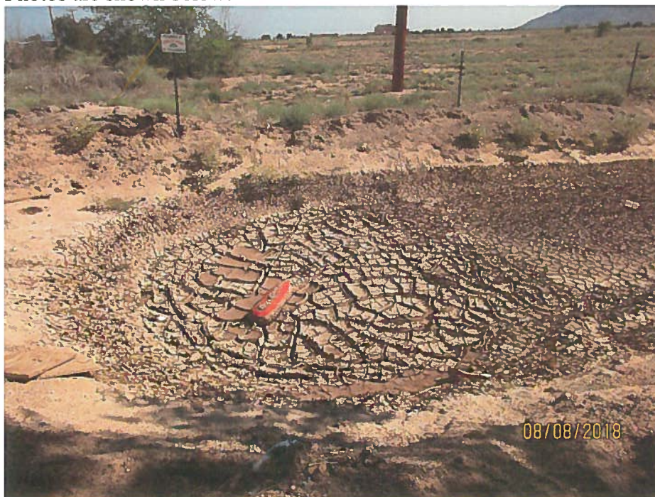
Inlet grate buried under sediment.
