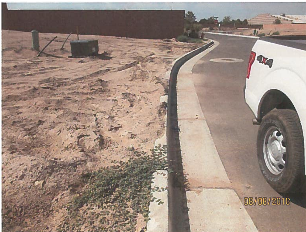
Sediment BMP (cut-back) needs improvement on this lot.
