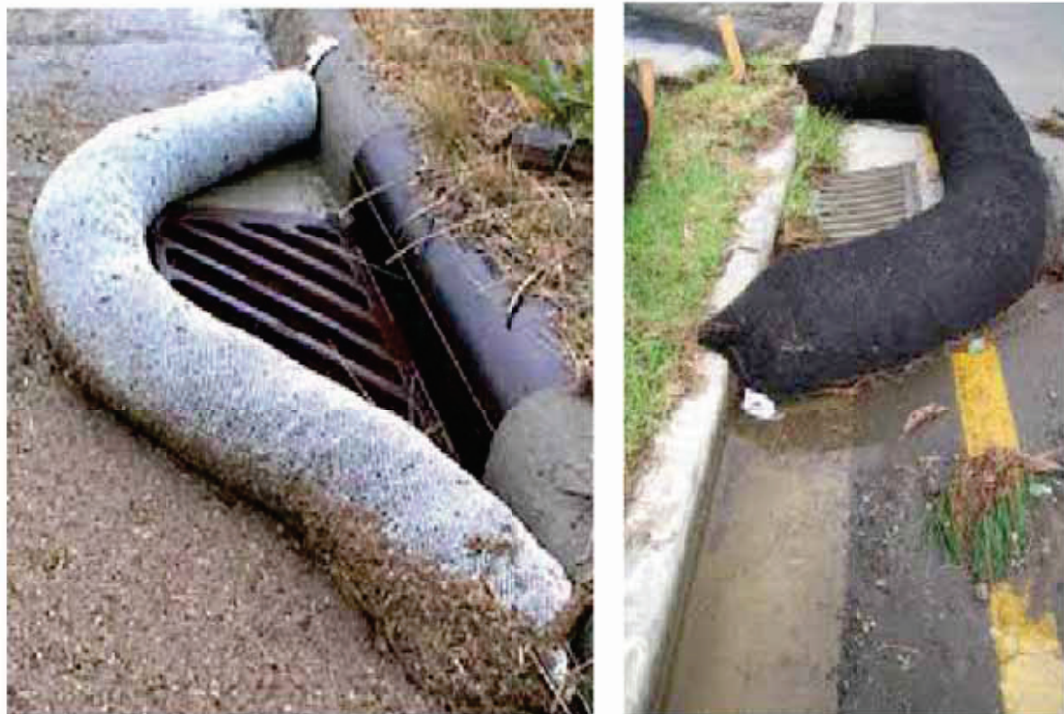
Curb Storm Inlet Protection with Wattles
