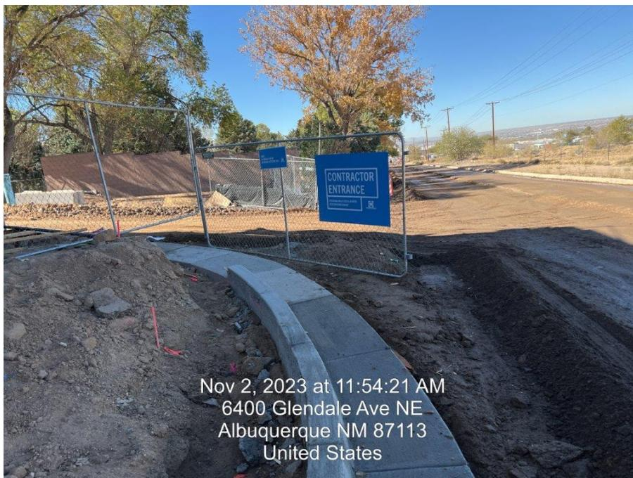
3. **Sediment** has been tracked out the two entrances into the paved portion of Glendale Ave. north and west of the site, where excess water from the water truck was flowing from the site down to the City's existing storm drain at San Pedro Dr.
