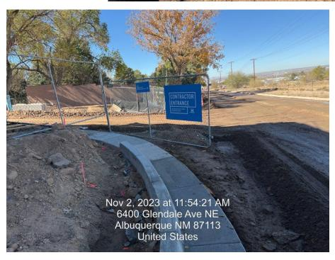
3. **Sediment** has been tracked out the two entrances into the paved portion of Glendale Ave. north and west of the site, where excess water from the water truck was flowing from the site down to the City's existing storm drain at San Pedro Dr.
