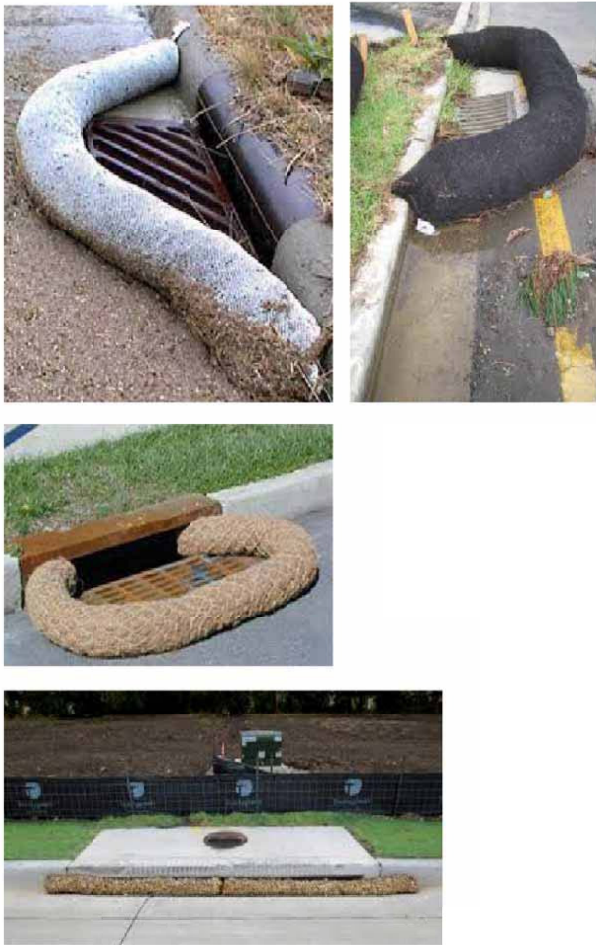
Curb Storm Inlet Protection with Wattles
