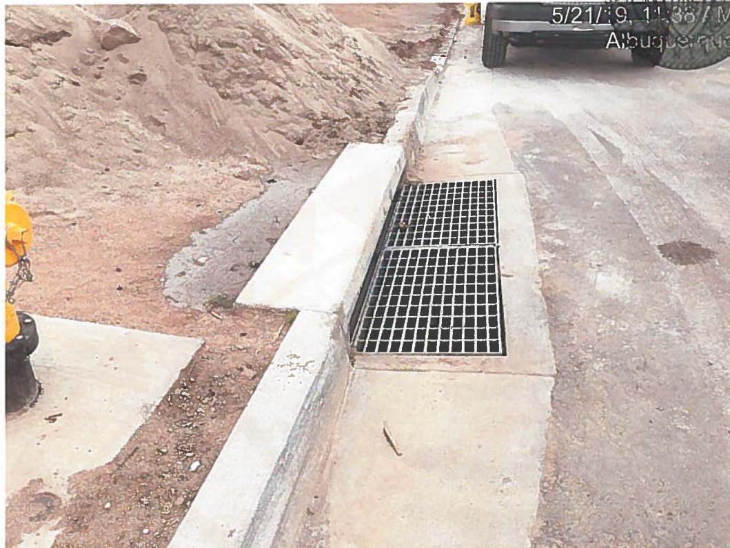
No inlet protection, no BMP for sand pile and wash-out in the dirt.
