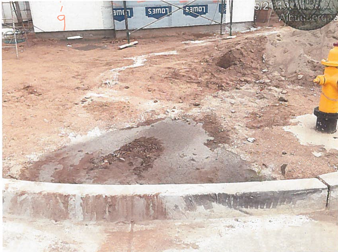
9119 Moon Dust: Wash-out in the dirt and in the gutter
