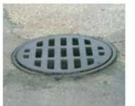
Remove sediment, debris, ice and snow from the inlet grate surface and surrounding area.
