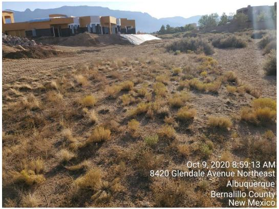
2. The disturbed area and construction activities overlap with construction support activities on the adjacent property at 8500 Glendale, owned by John Jones which also requires NPDES coverage. The SWPPP must identify the areas of control by each Operator.
