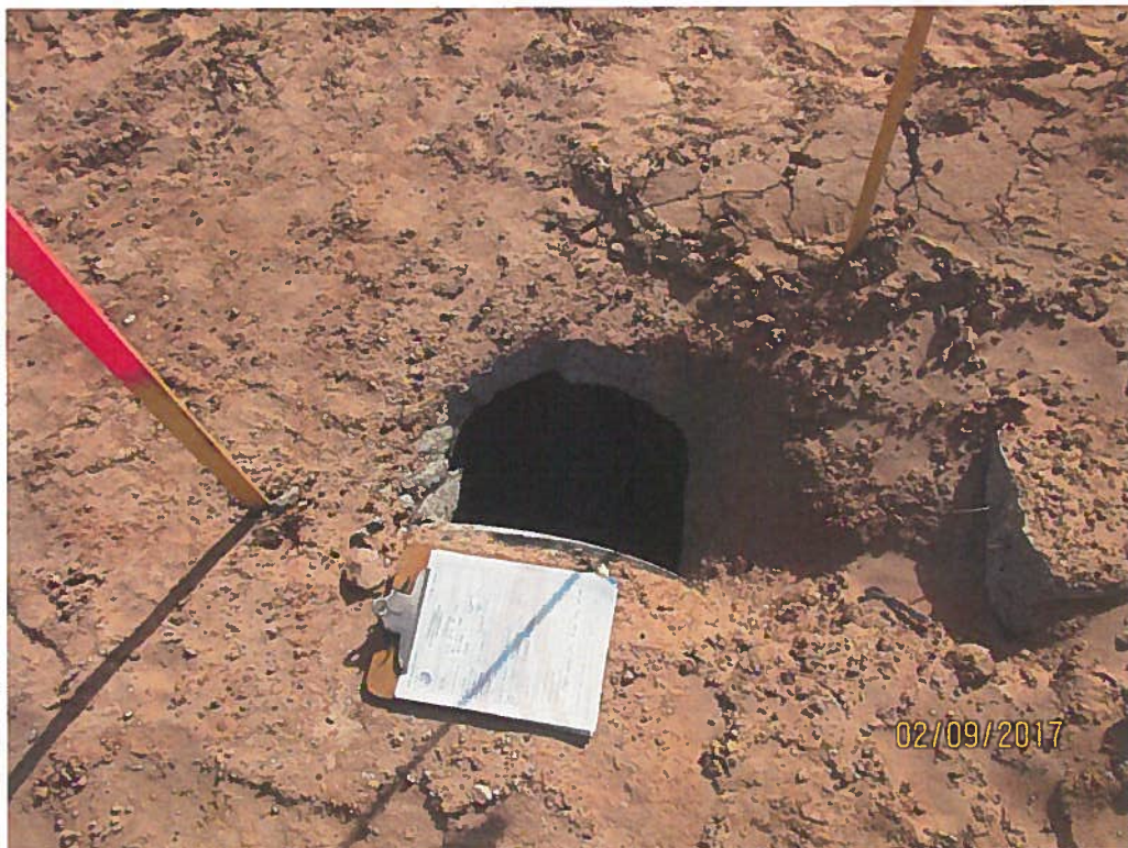
Opening in storm drain caused by contractor.
