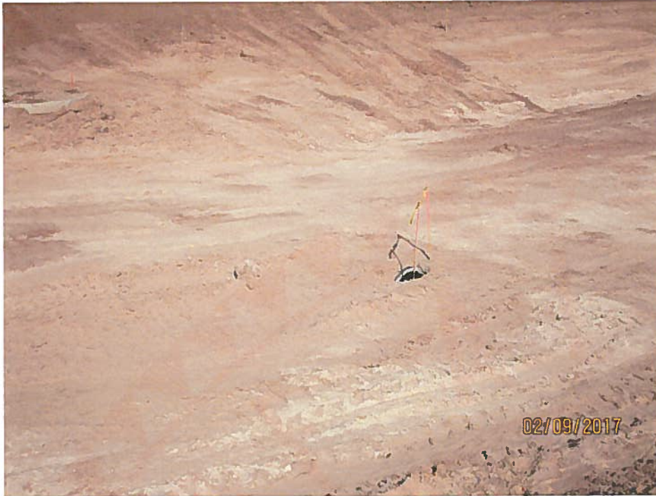
Opening in storm drain showing location in bottom of pond.
