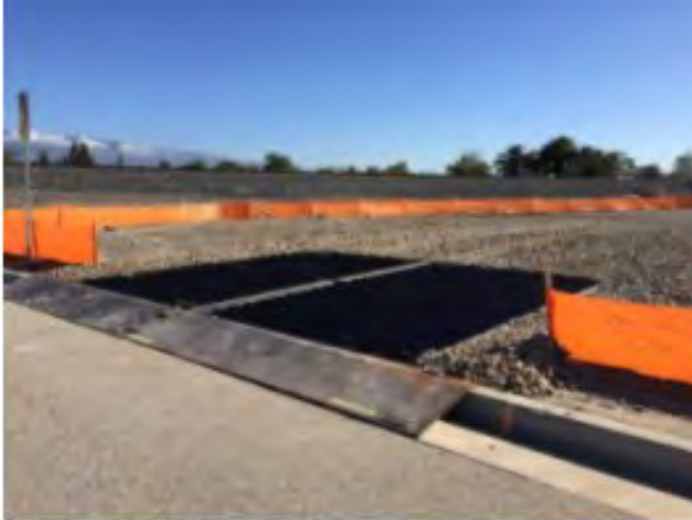
SEDIMENT TRACK OUT CONTROL
