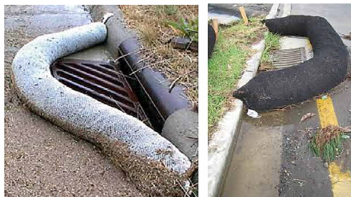
Curb Storm Inlet Protection with Wattles
