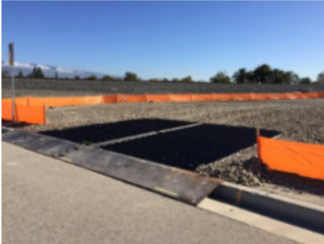
SEDIMENT TRACK OUT CONTROL
