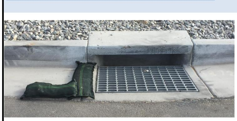
Inlet gravel bags are manufactured on site to fit in the gutter pan on the upstream side of the inlet. Filled with smooth rounded pea gravel. The ends are sealed with  $\frac{1}{2}$ " #12 hog rings. The gravel bags are connected together with the hogs to help create weight and stability.
