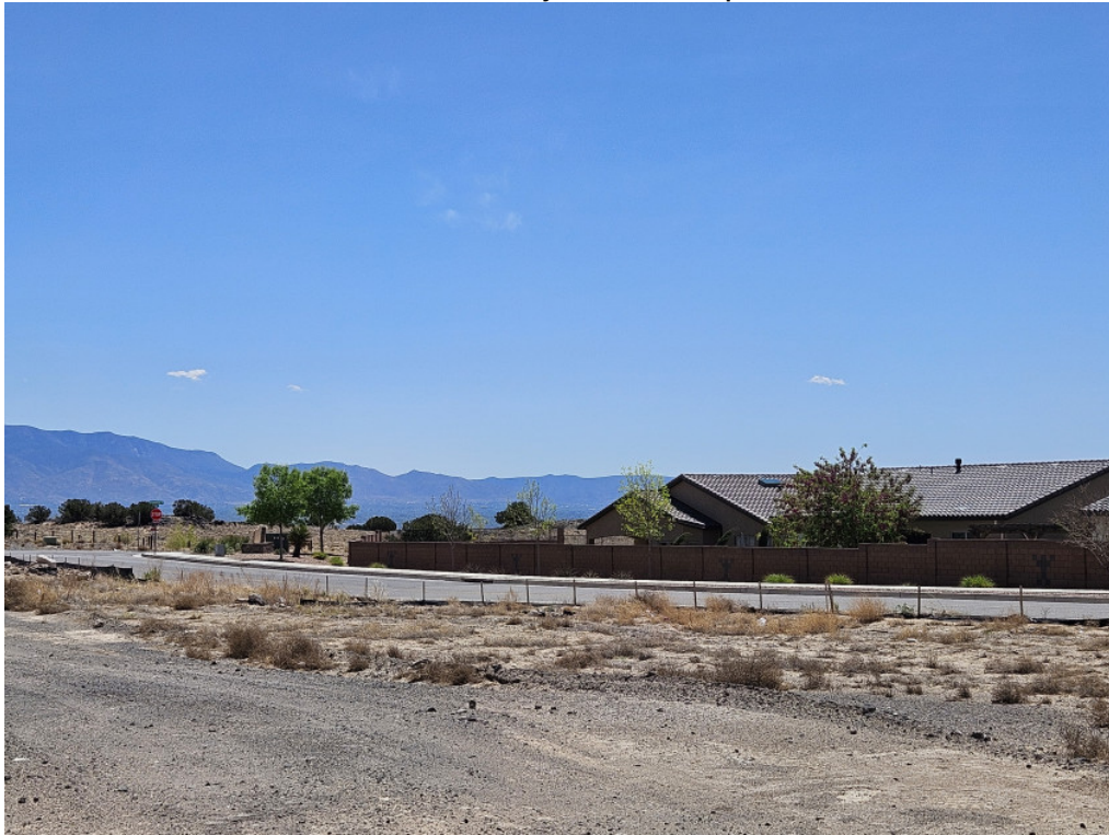
Site Walk Deficiency Photos - Rosa parks
