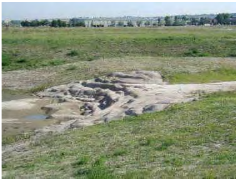
Photo 1: Sculpted Shotcrete Grade Control Structure
