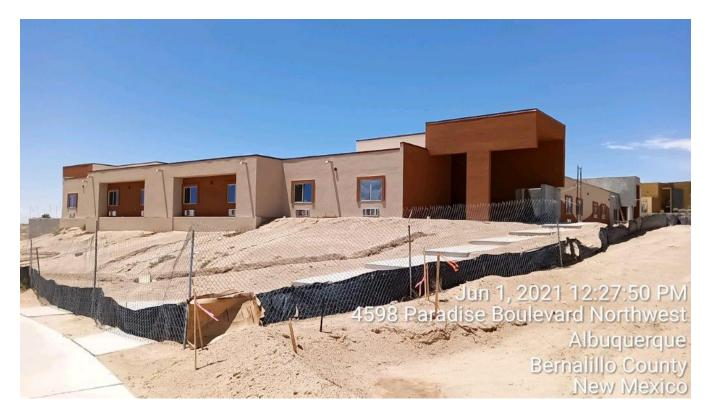
3. Sediment washed into the street and sidewalk during the rain on 5/31 and was not cleaned up on 6/1.
