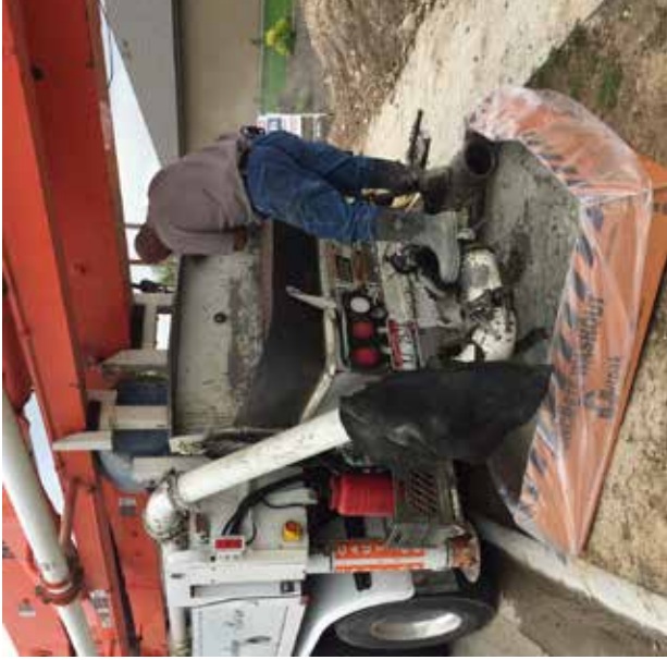
6x6 Outpak Pump Washout holds up to 1.3 cubic yards of concrete and waste water.
