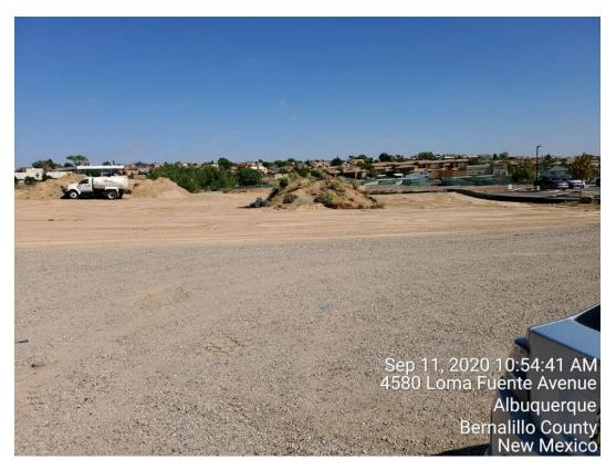
2. BMPs are mostly missing or in need of maintenance. The Construction Entrance, sediment trap, and most of the silt Fence are missing. The existing Silt Fence needs maintenance.
