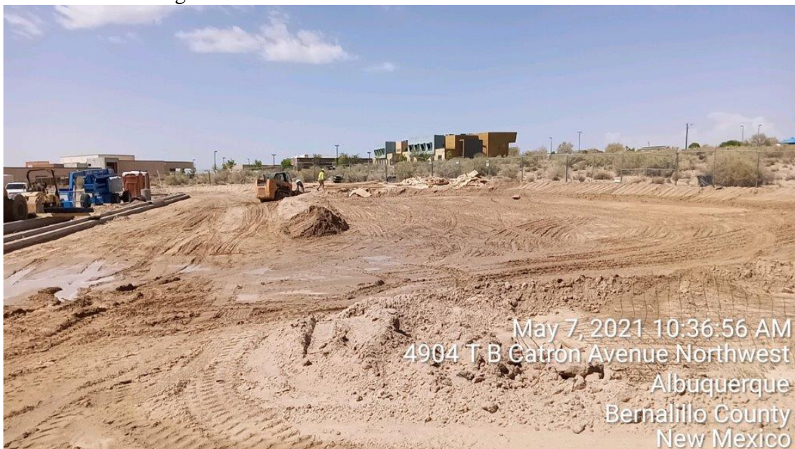
Silt Fence is missing west side of site
